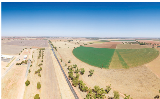
Parkes to Narromine section of Inland Rail, New South Wales
