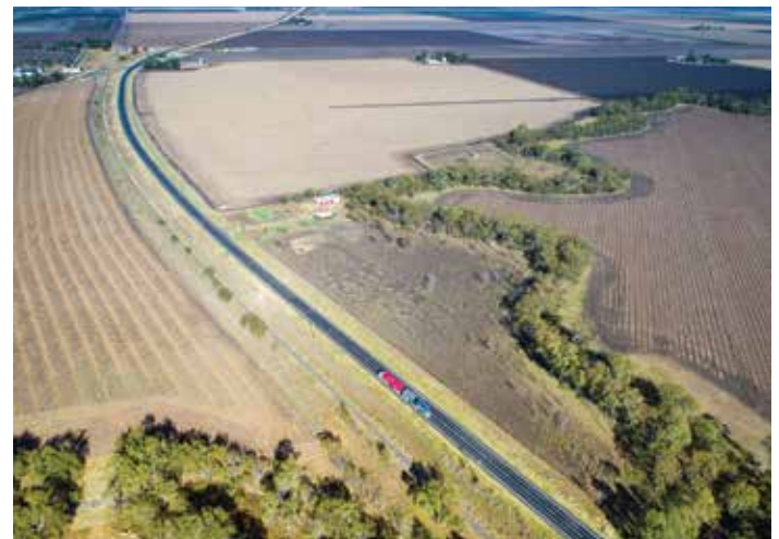
The existing railway line, Gore Highway, Pampas.
