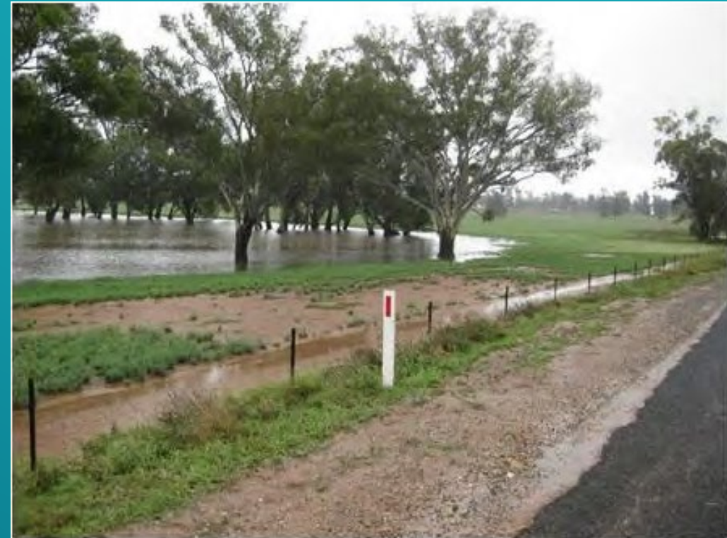
Flooding at Ulandra Creek near Ironbong Road
