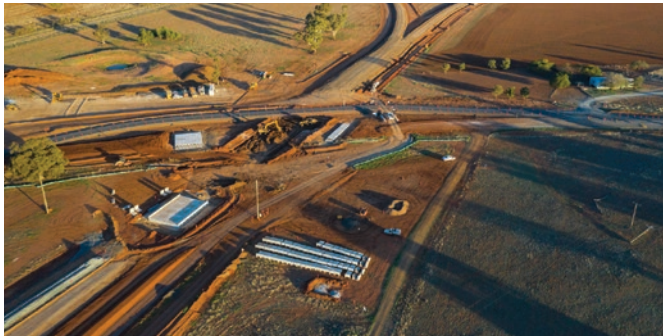
North West Connection work under way
