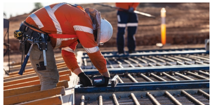
Installing drainage structures, P2N project
