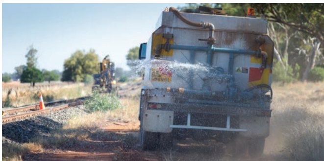
Water truck to minimise dust
