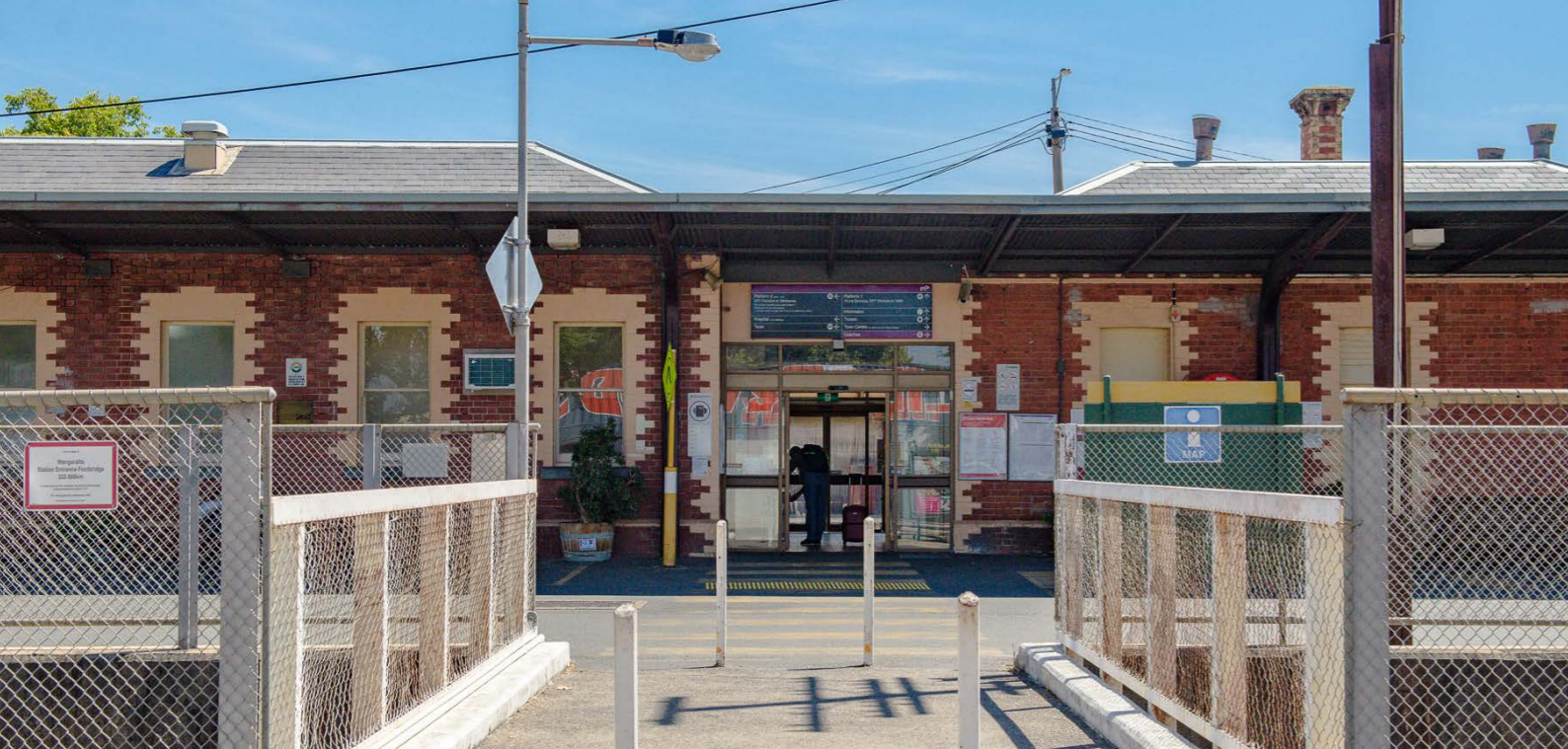
Wangaratta Station, Wangaratta
