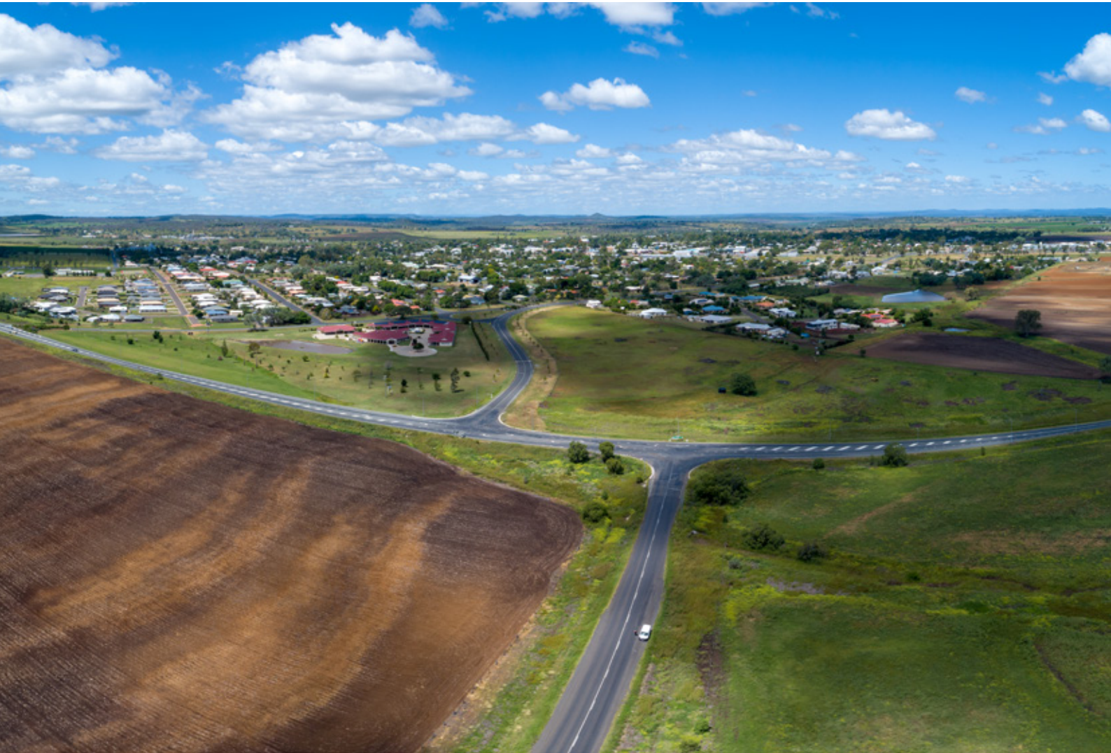
Gore Highway near the township of Pittsworth
