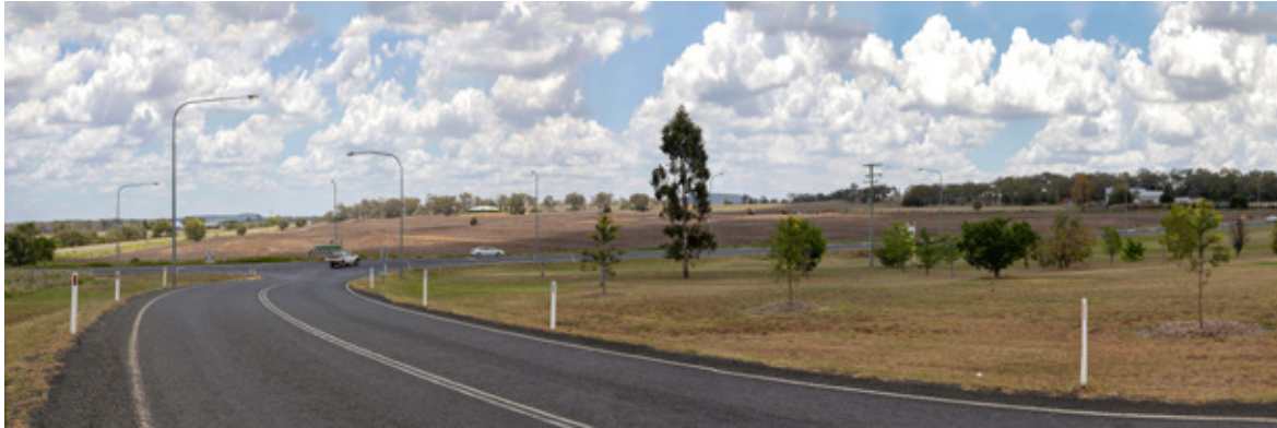
Pittsworth Felton Road, Pittsworth, looking north west towards Oakey-Pittsworth Road and the Gore Highway (current)
