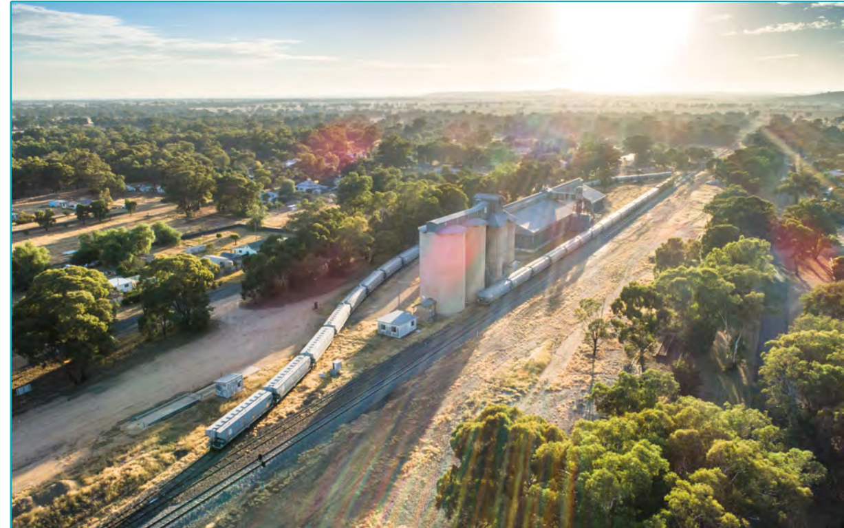
Existing rail infrastructure in Stockinbingal
