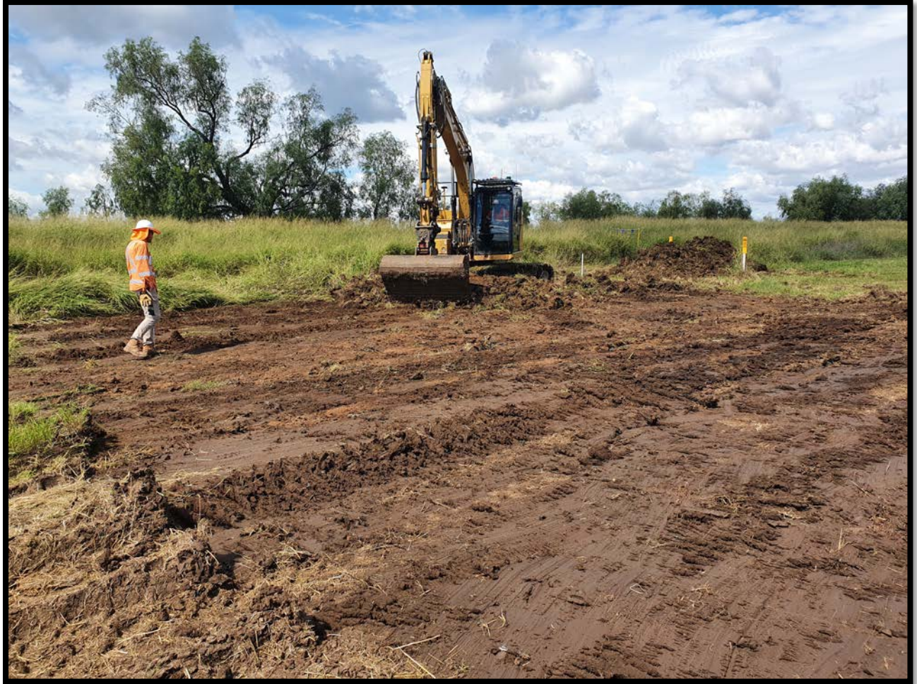
Plate 5-4. Example of top soil stripping to 100 mm depth at 599.02 in Stage 1.
