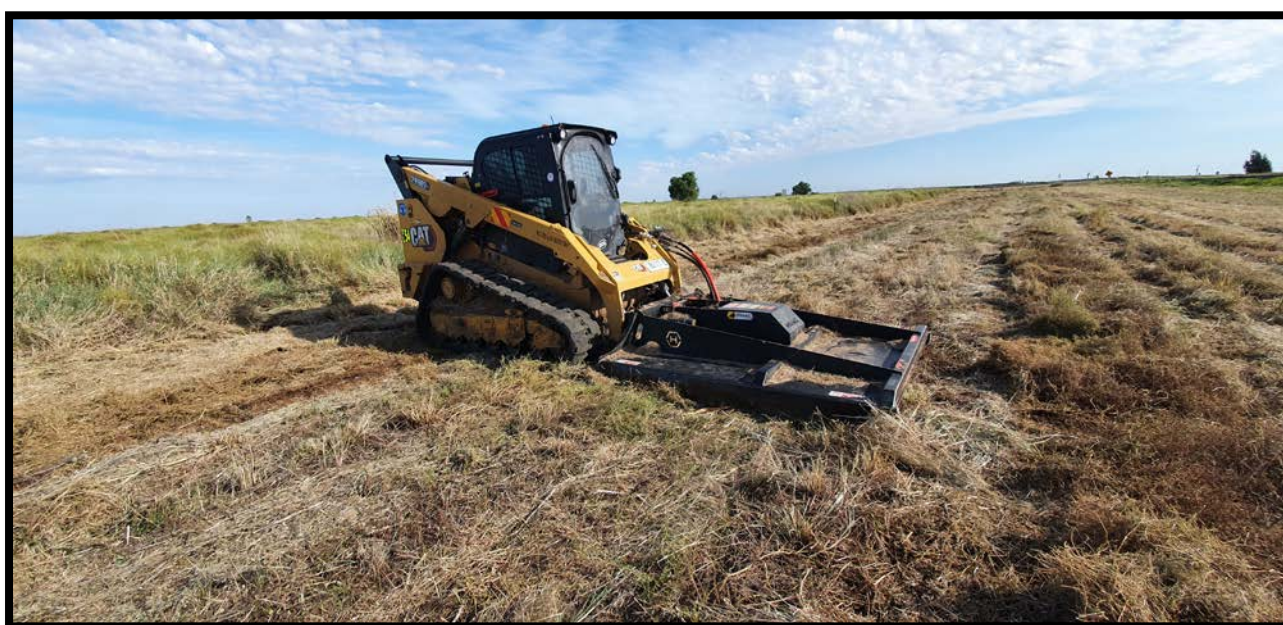
Plate 5-2. Slashing on vegetation prior to stripping in Stage 1.
