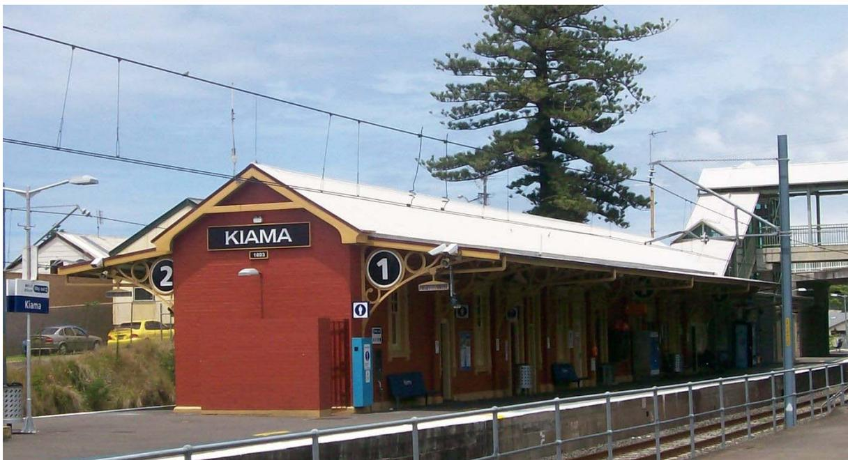
8. View of Kiama Station showing an alternative two-platform design necessitating a footbridge (Type 11). Ornate brackets are on both platform awnings with intrusive platform number labels (see image 9) (source: WikiCommons).
