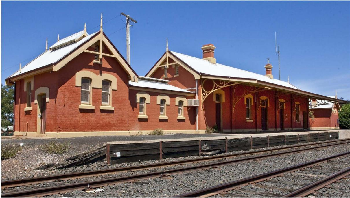
3. View of platform at Cobar Station. Note asphalt platform and timber platform edge coping. Awning brackets are in yellow, in contrast to the red/brown finish at Parkes, Temora, and Forbes. Orientation of men's toilet (left) is reverse to that at Forbes. (Source: WikiCommons)
