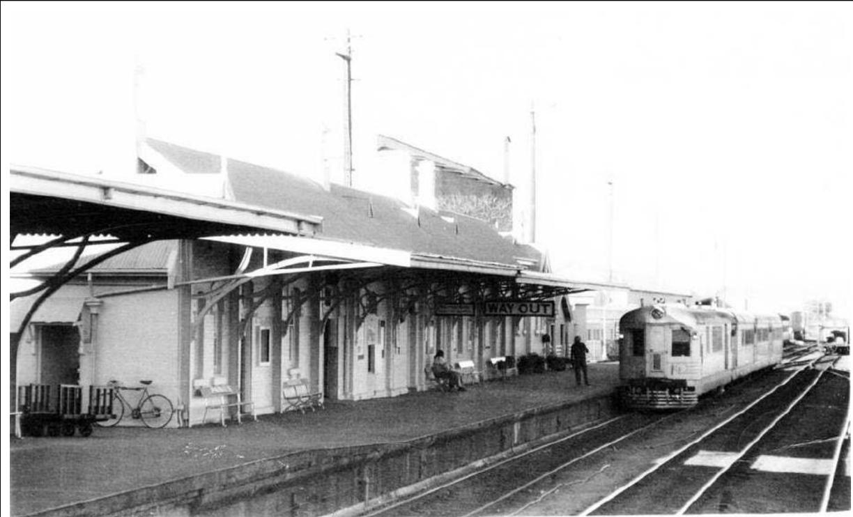
1. View of Parkes Station showing the edge of western station building awning (left) and eastern (original) Type 4 station building to the right. Note the difference between the ornate brackets used on the building to the right and the simple brackets on the building to the left (source: Parkes Champion Post, date unknown).
