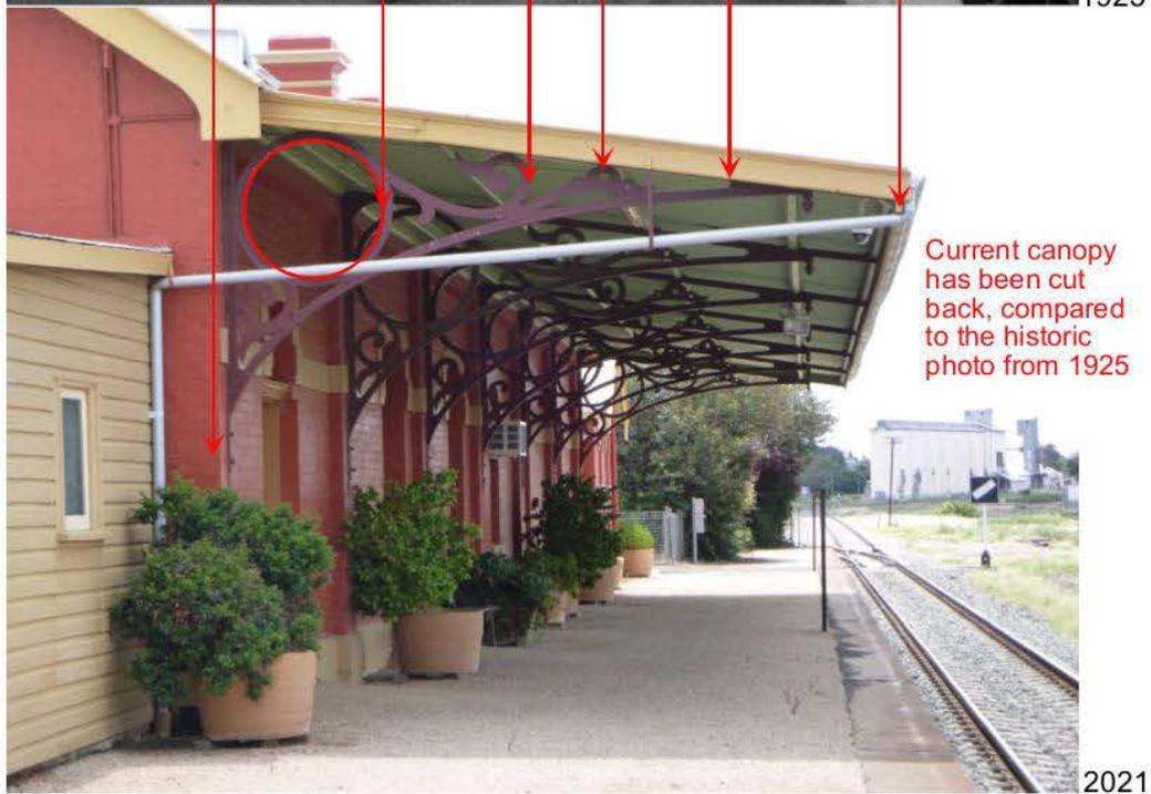
Photo of underside of existing Station Canopy
