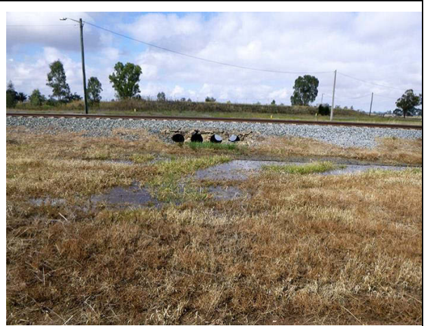
2. View of the disturbances in the Bribbaree yard, culverts and previous construction of the railway line.
