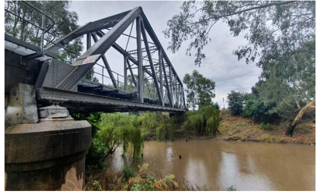
Photo 4.6 Lachlan River Bridge
