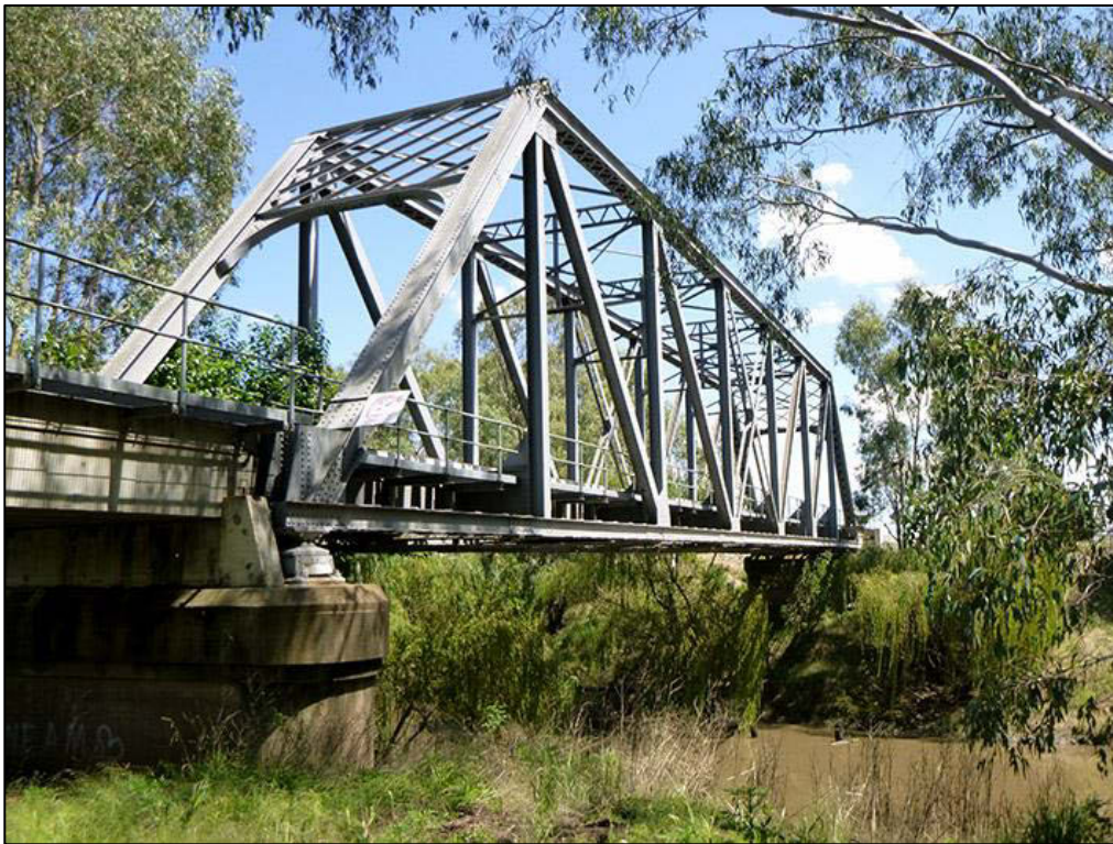
View to the northwest showing the Lachlan River Rail Bridge.
