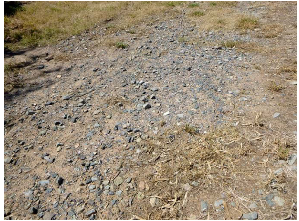
View of the railway ballast screed across the ground surface.
