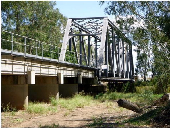
View to the northwest of the Lachlan River Bridge showing ground disturbance from bridge construction.
