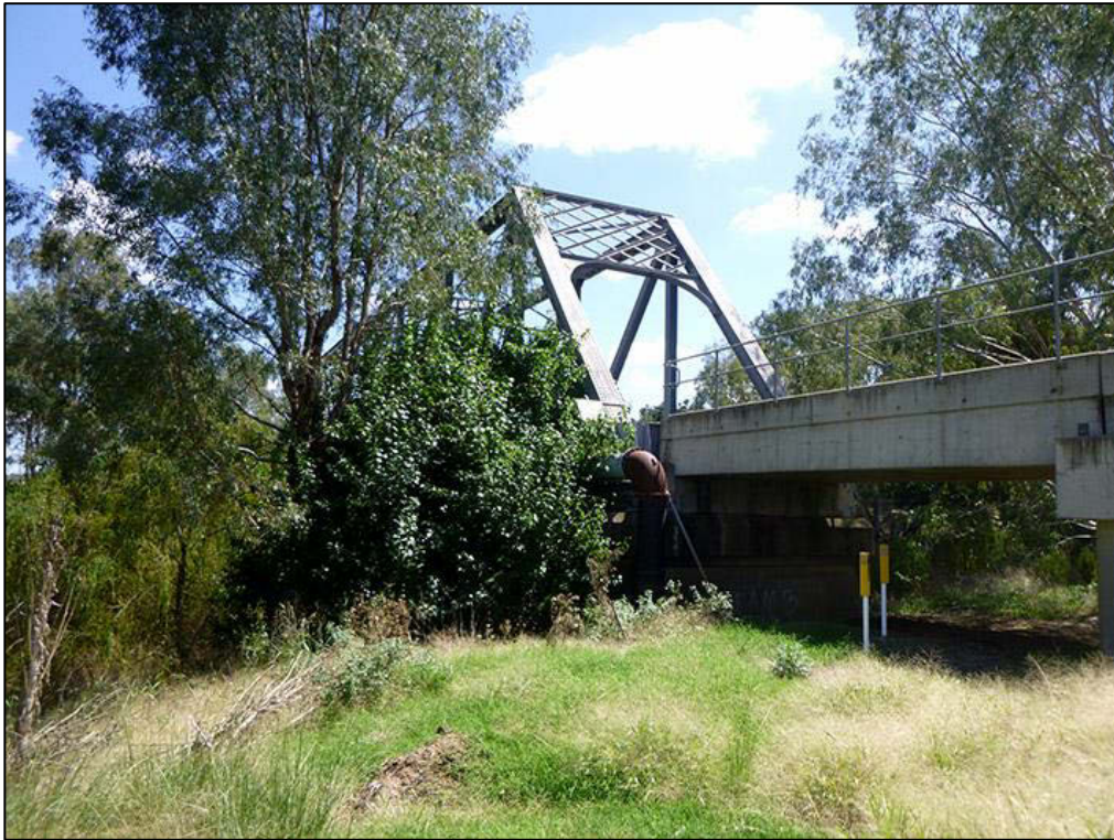
Plate 3: View to the northeast showing the bridge and railway infrastructure that has caused ground and sub surface disturbance directly adjacent to the Lachlan River.
