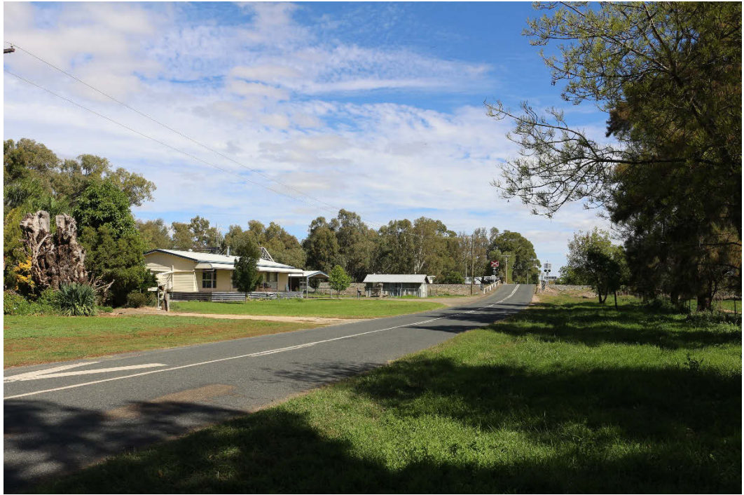
FIGURE 5-1 VIEW SOUTHWEST FROM LOWER BATHURST STREET TOWARDS THE PROPOSAL SITE
