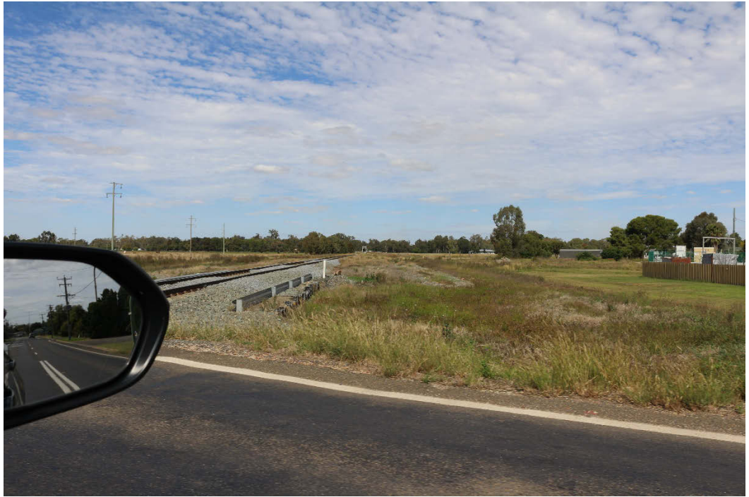
FIGURE 5-5 VIEW SOUTHEAST FROM ESCORT WAY ALONG THE RAIL CORRIDOR TOWARDS THE PROPOSAL SITE
