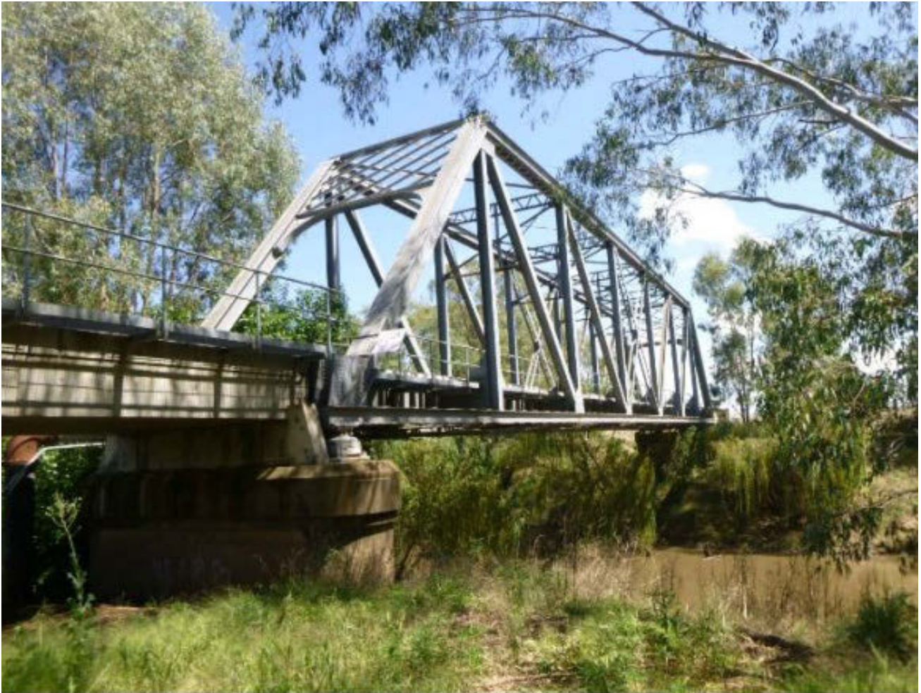
Figure 1.1 Existing Lachlan River Bridge truss structure from the south
