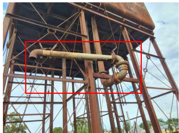
FIGURE 2.6 QUANDIALLA WATER TANK, SHOWING PIPEWORK EXTENDING FROM FRAME (SEE RED OUTLINE)
