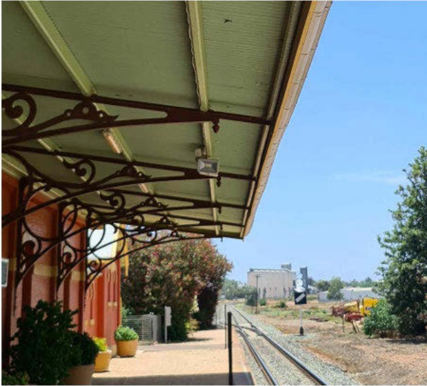
FIGURE 2.7 PHOTO OF AWNING AT FORBES STATION
