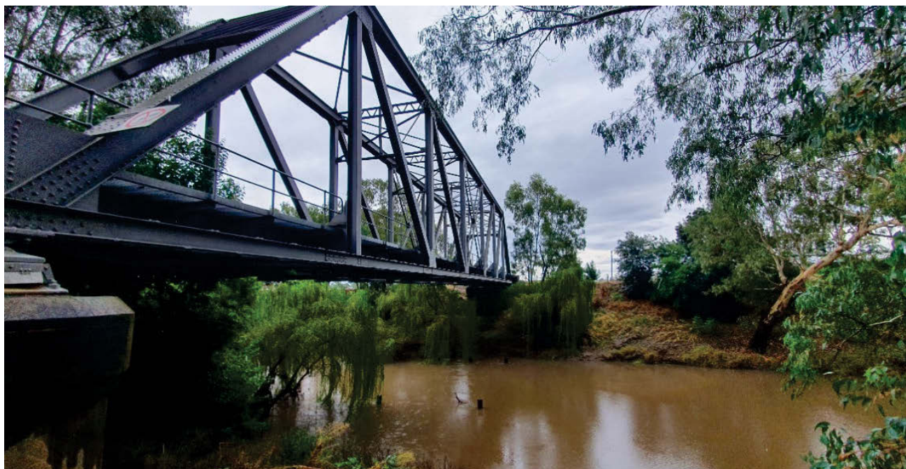
FIGURE 5.6 LACHLAN RIVER BRIDGE AND LACHLAN RIVER
