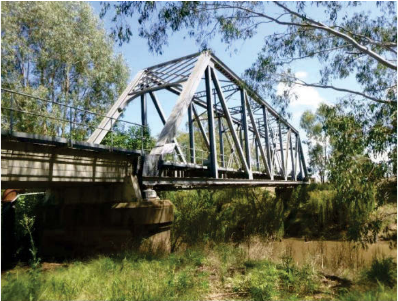
FIGURE 2.2 EXISTING LACHLAN RIVER BRIDGE TRUSS STRUCTURE FROM THE SOUTH
