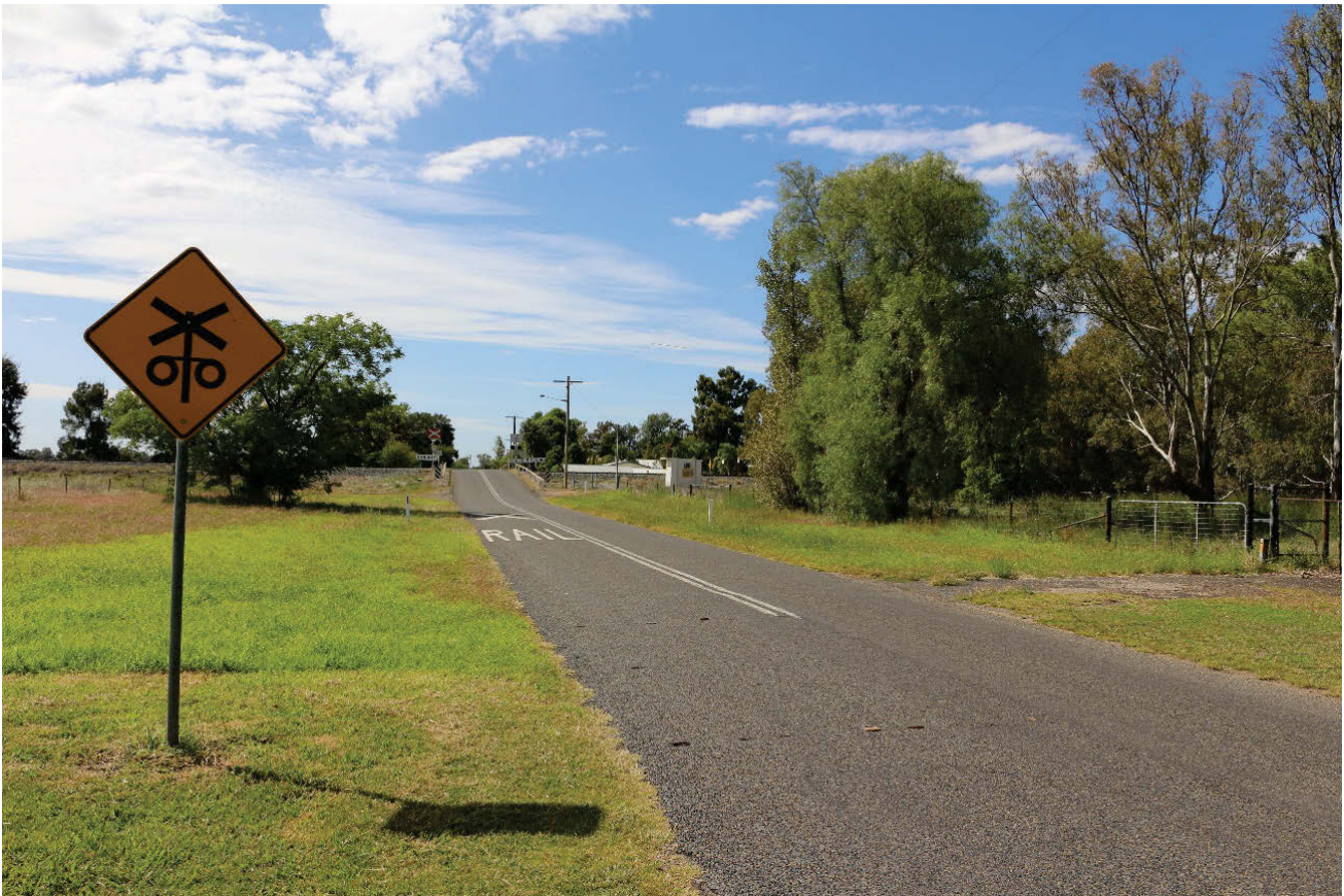
FIGURE 5.15 PHOTO OF THE LEVEL CROSSING ON BATHURST STREET FROM THE WEST
