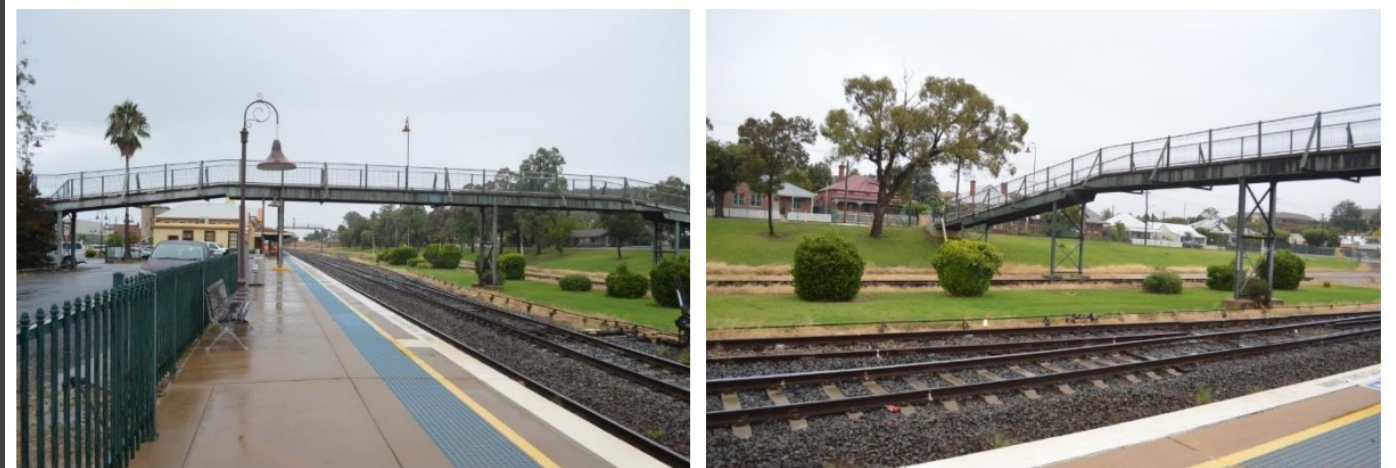
Figure 40 'Mother's Bridge' footbridge within the Wagga Wagga Railway Station yard.
