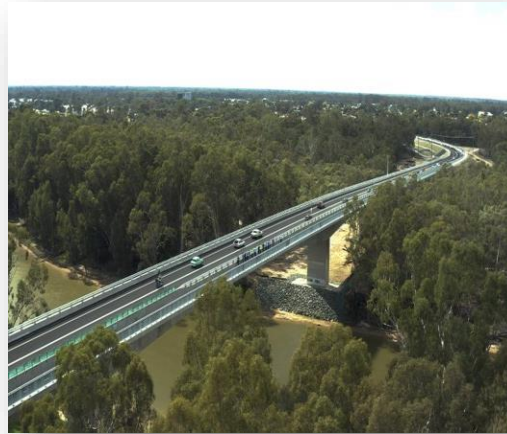
Echuca Moama bridge
