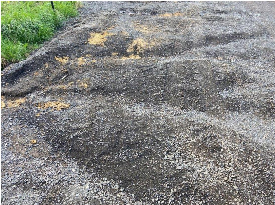
Plate 30 – 10 Mile Creek Bridge evidence of pad erosion
