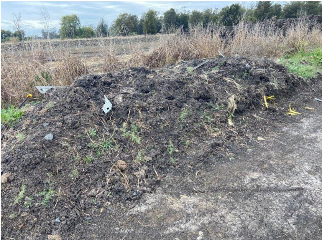
Plate 38 – Yallaroi laydown stockpile contaminated with foreign materials
