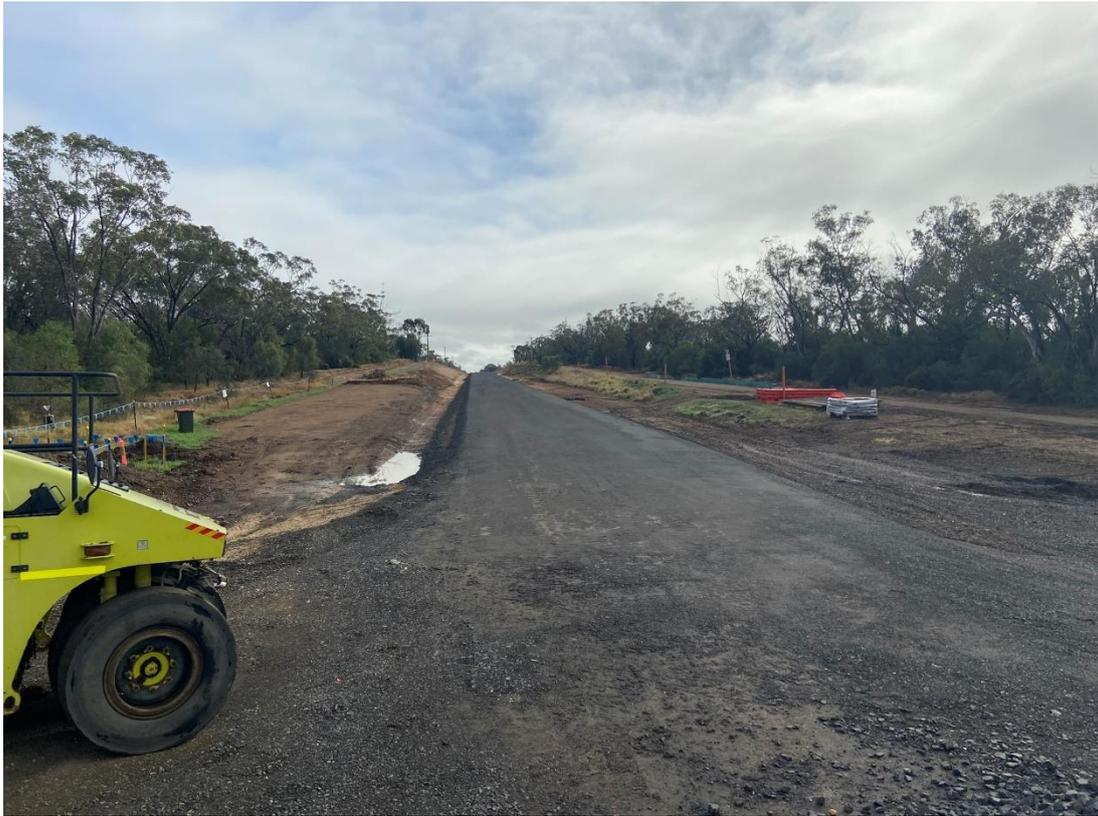
Plate 3 – Subgrade installed in alignment
