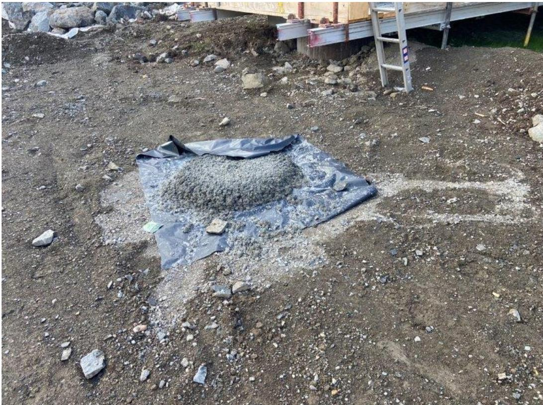
Plate 32 – 10 Mile Creek concrete spillage on piling pad
