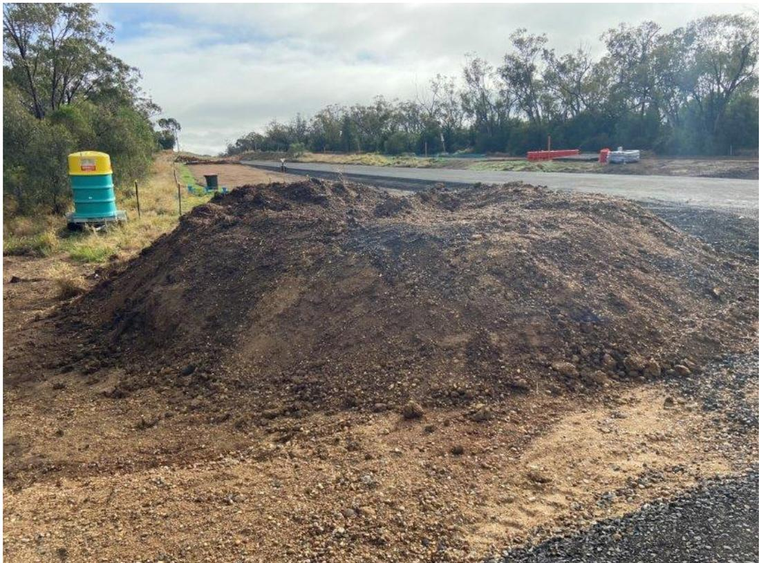
Plate 4 – Temporary stockpile not adequately managed in accordance with SWMP
