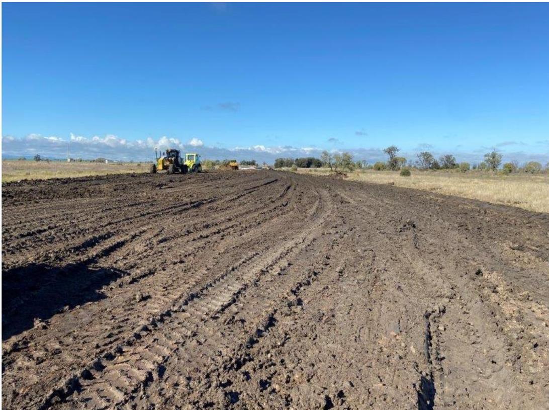
Plate 10 – Bellata CH614.77 muddy condition along alignment
