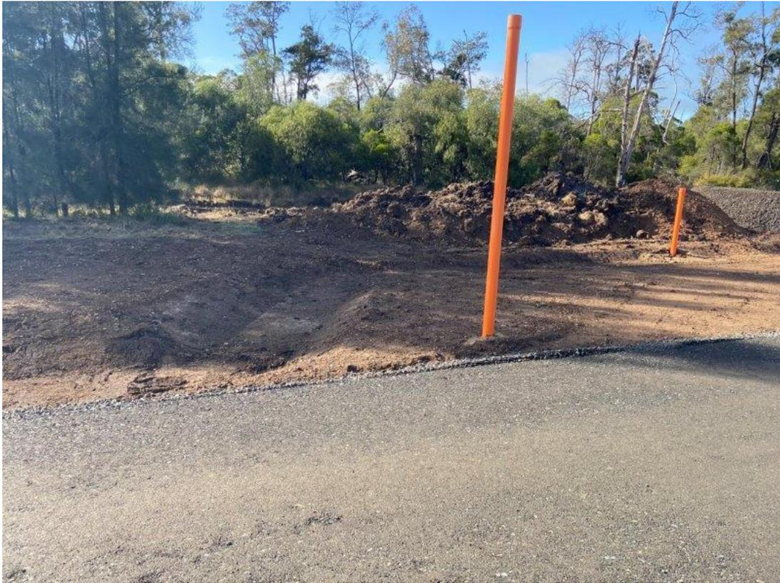
Plate 9 – Temporary stockpile not adequately managed in accordance with SWMP along alignment CH621
