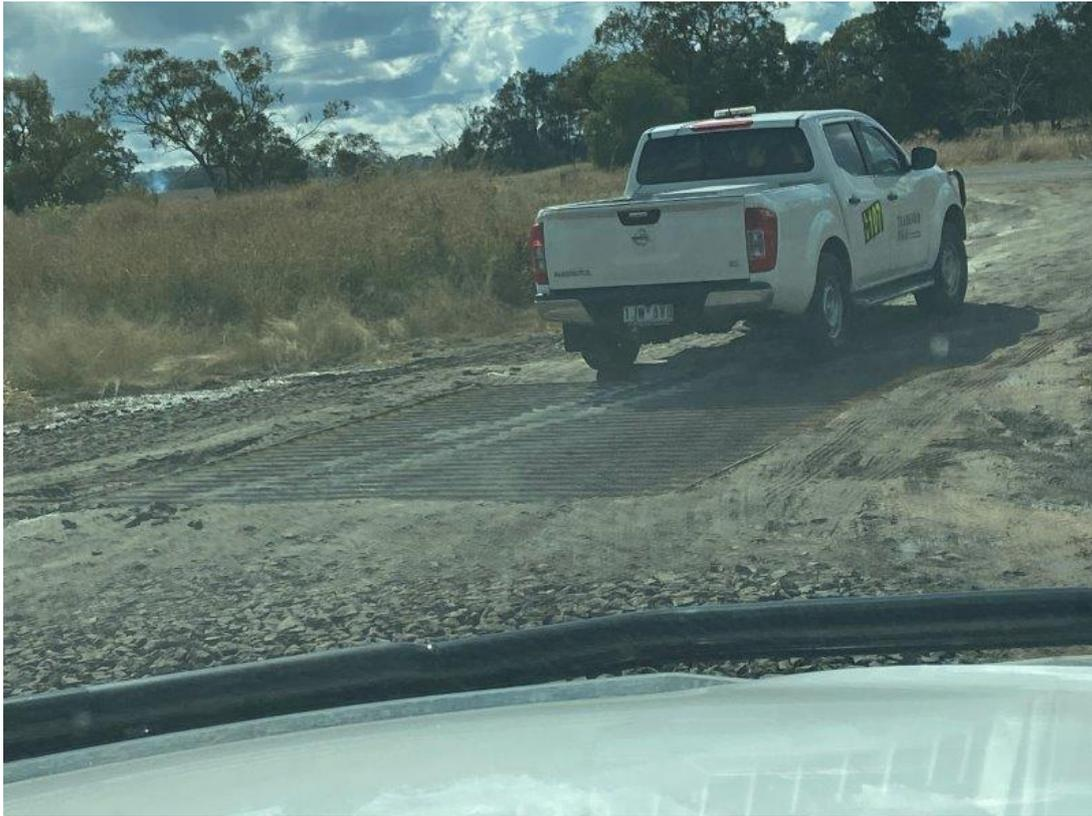
Plate 23 – Rumble grid utilised at Gate 7 MAF
