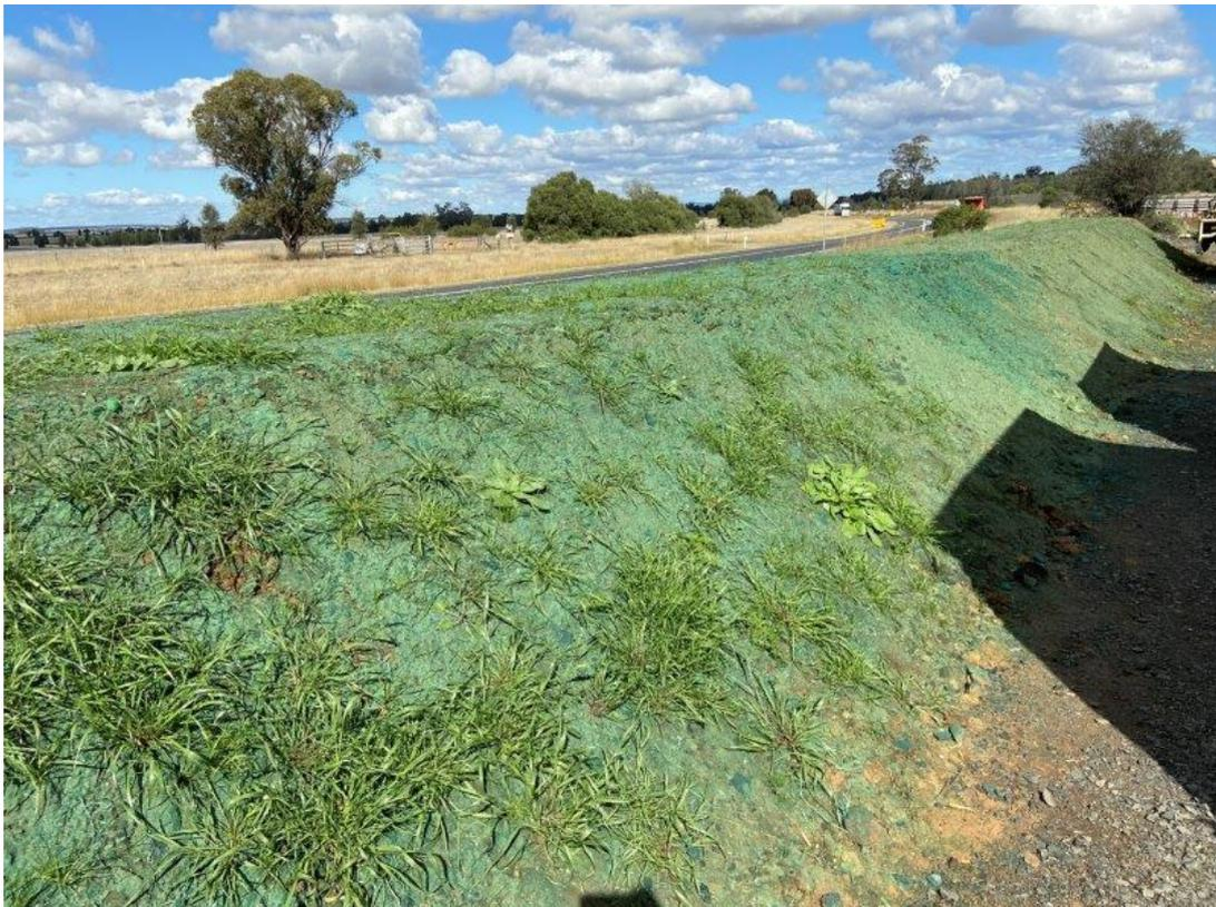
Plate 24 – Spray grass applied to batter
