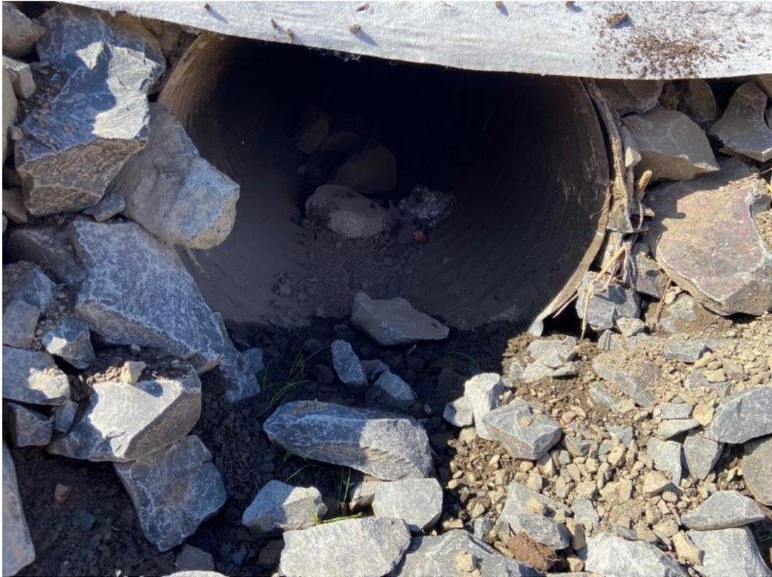
Plate 27 – Bobbiwa Bridge minor material located within pipes
