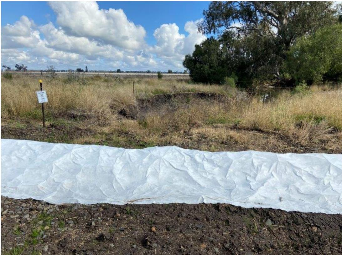
Plate 22 – Sediment control structures within CIZ along with signposting at Gate 7
