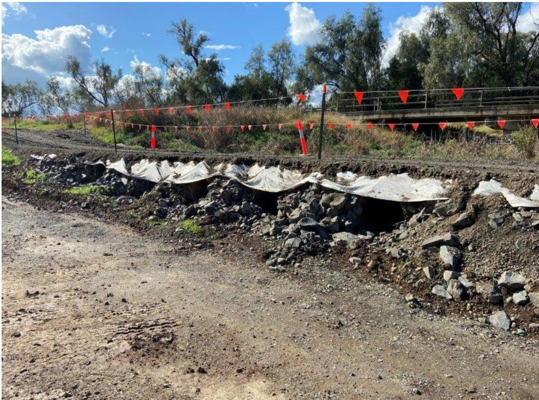
Plate 26 – Bobbiwa Bridge evidence of erosion of rock protection
