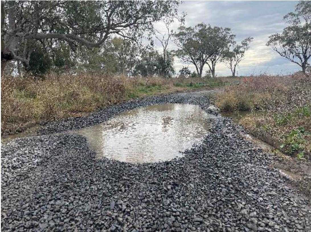
Plate 37 – PAD 2 Gurley Bridge causeway with indications of sediment migration and erosion downstream
