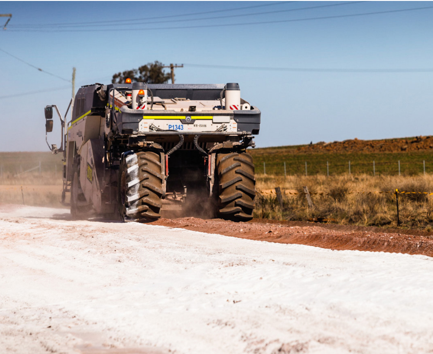
The lime stabilisation process in action
