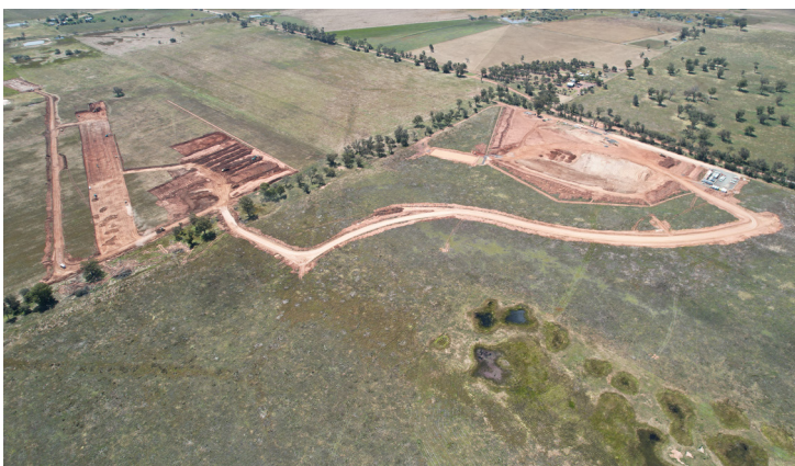
Aerial view of Narwonah MDC showing progress on the earthworks
