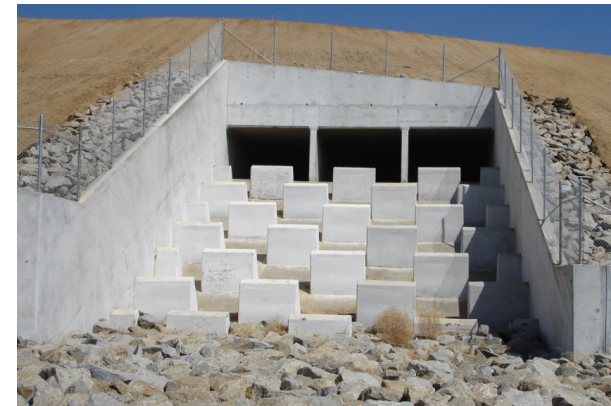
Energy dissipater to reduce velocities
