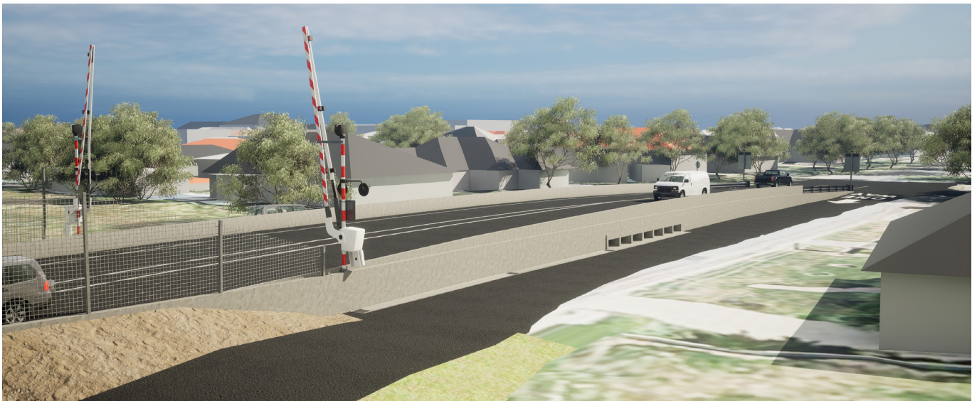
Visualisation of the Anderson Street proposed road underpass showing the flood and safety mitigations required at the southern entry
