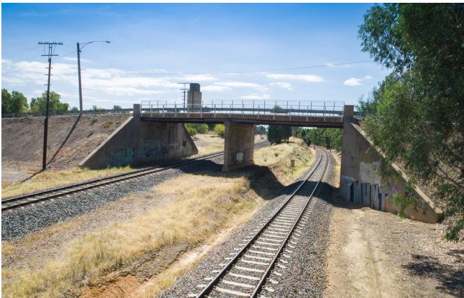
Existing Green Street bridge.
