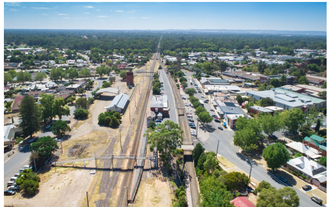
Existing Wangaratta Station.
