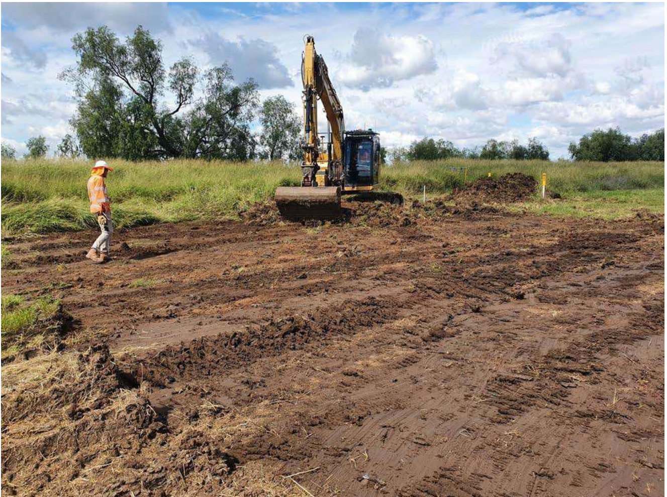
Figure 6-3: Example of topsoil stripping to 100 mm depth at N2NS SP1
