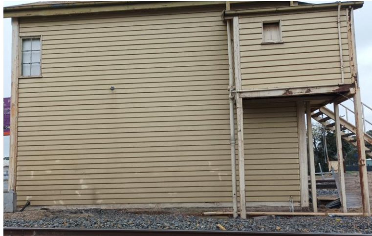
Figure 3-6: General condition of steel weatherboard cladding
