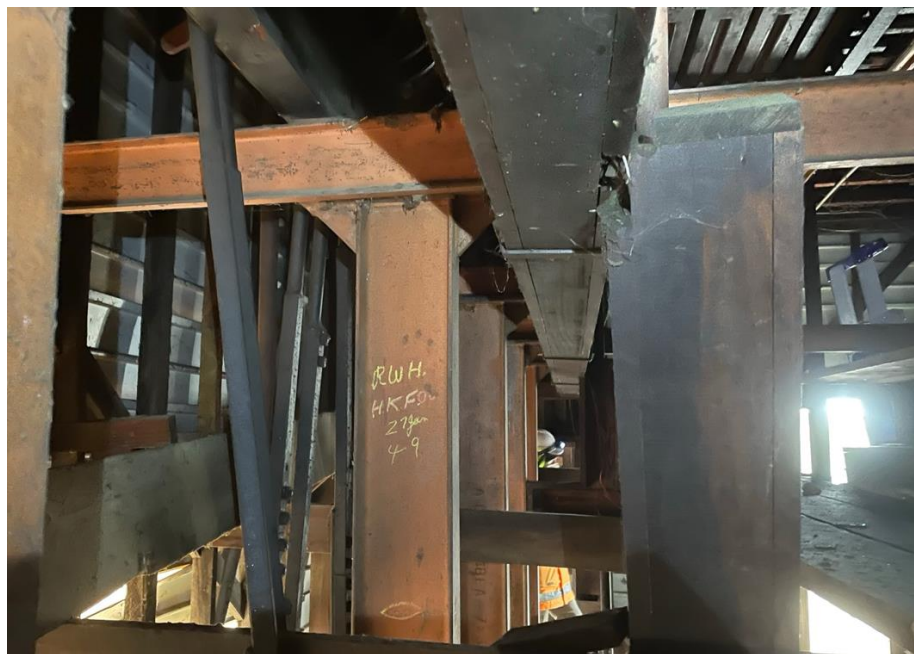
Figure 3-41: Internal steel lever frame supports
