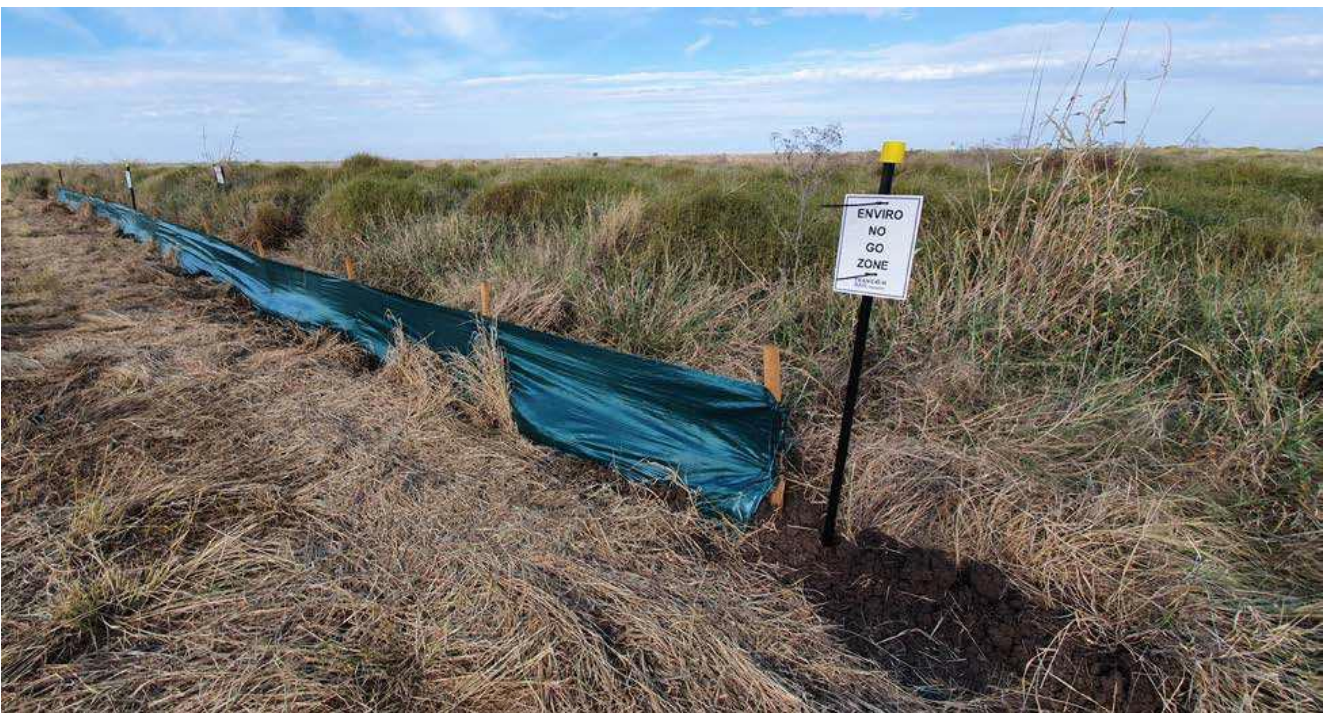
Figure 6-2: Example of a FCWS relocation hub installed at N2NS SP1 supported by environmental signage
