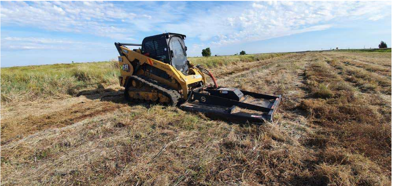
Figure 6-1: Slashing of vegetation prior to stripping at N2NS SP1
