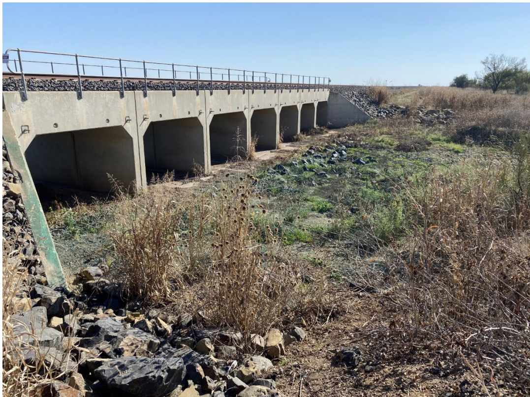
Plate 26 – Vegetation regrowth on eastern side of Bulldog Creek Bridge (operational)
