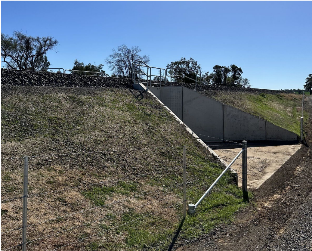
Plate 13 – Cattle underpass at CH745
