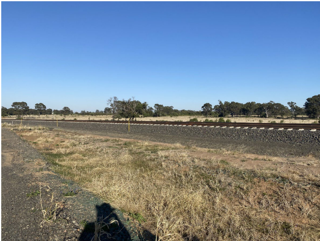
Plate 16 – Vegetation cover in drainage channel at Gate 2 (operational)
