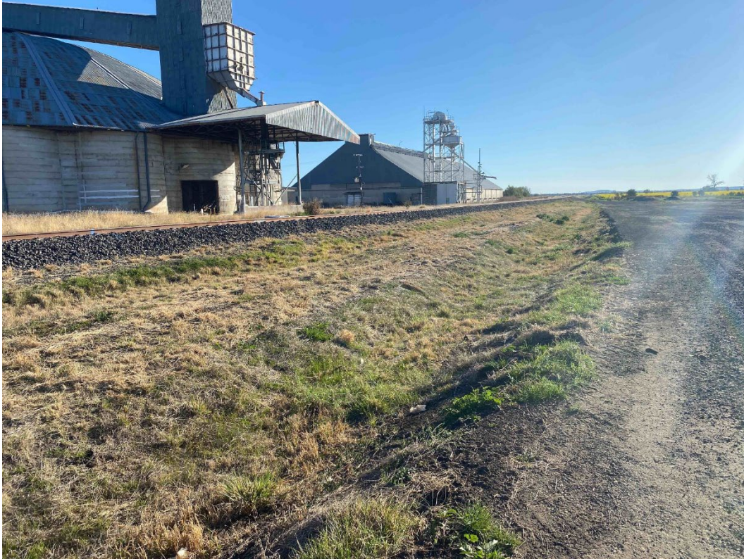
Plate 1 – Established vegetation cover in drainage channels next to Milguy Silos/Milguy MAF
