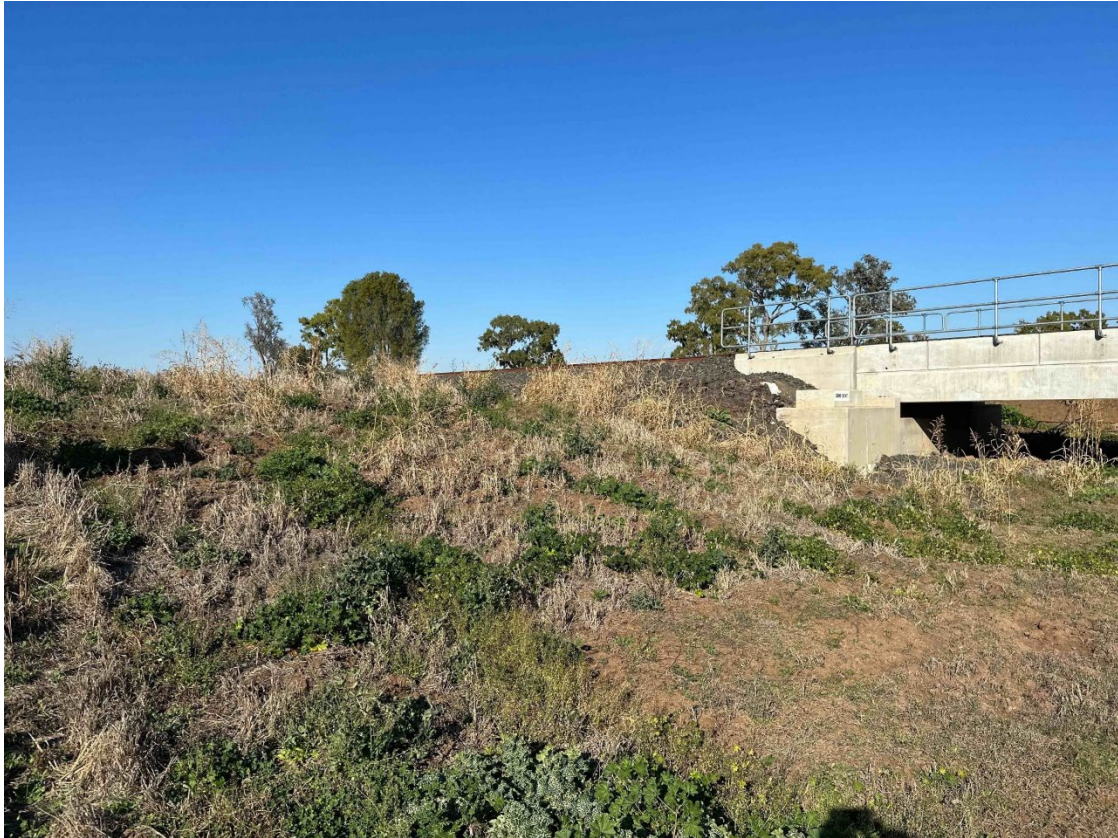
Plate 19 – Good vegetation cover with high weed presence along batters at Bobbiwaa Creek (operational)
