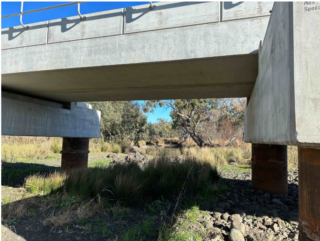
Plate 4 – Gil Gil Creek Bridge with dry waterbed
