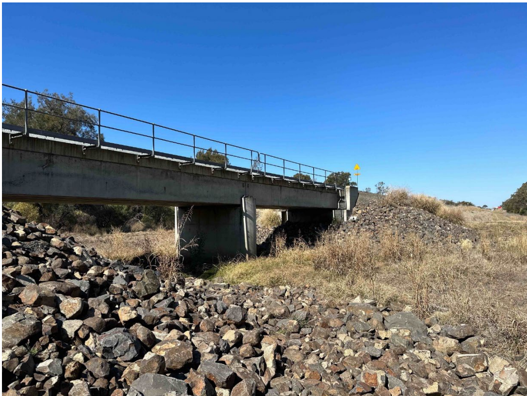
Plate 30 – Tookey Creek Bridge
