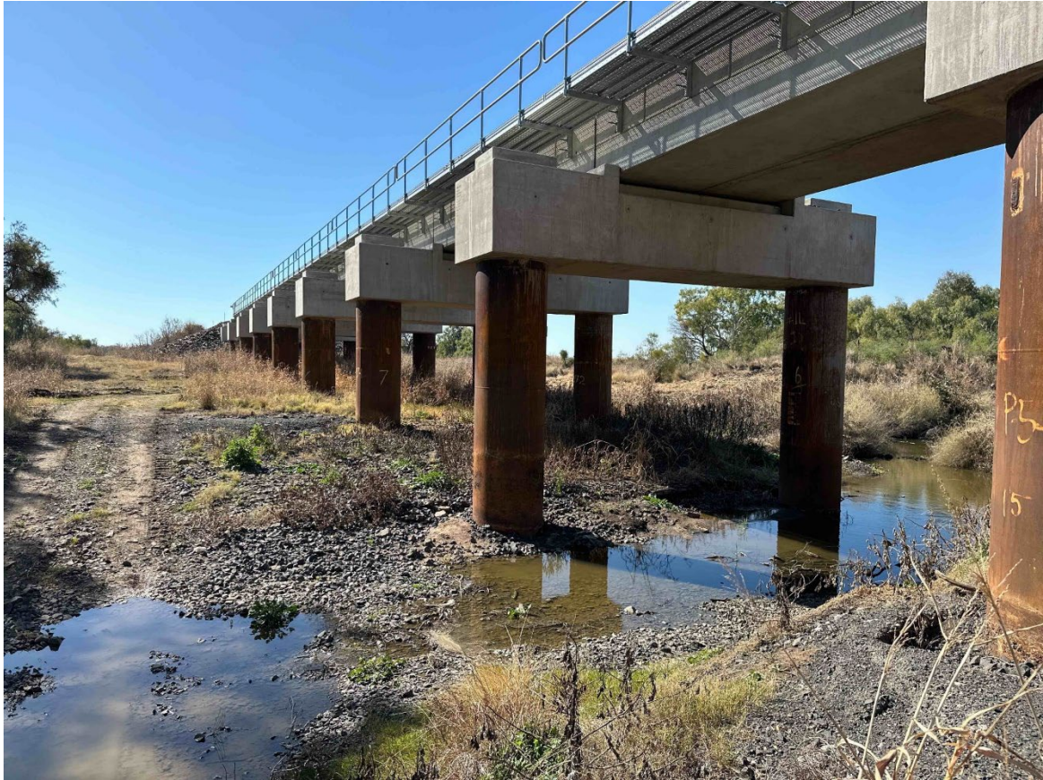
Plate 31 – Gurley Creek Bridge
