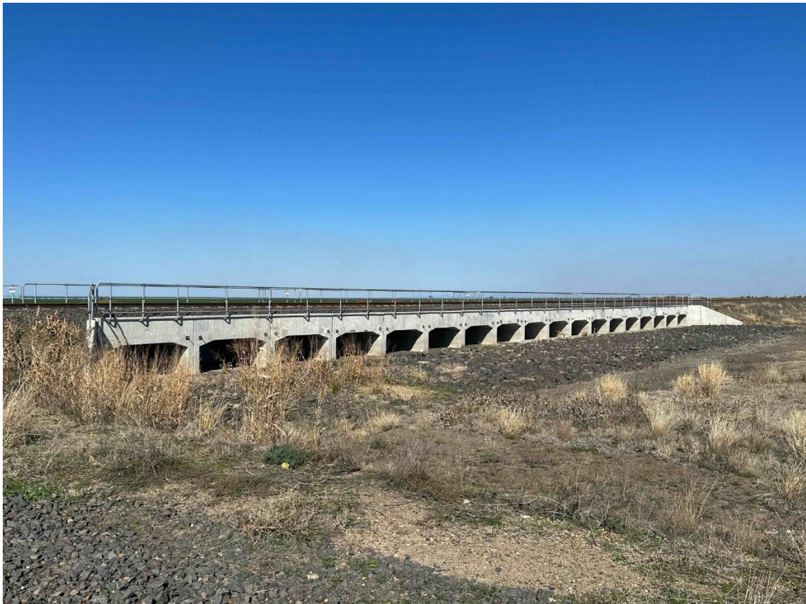
Plate 32 – Tycannah CH656 Culvert 500 with new rock scour protection
