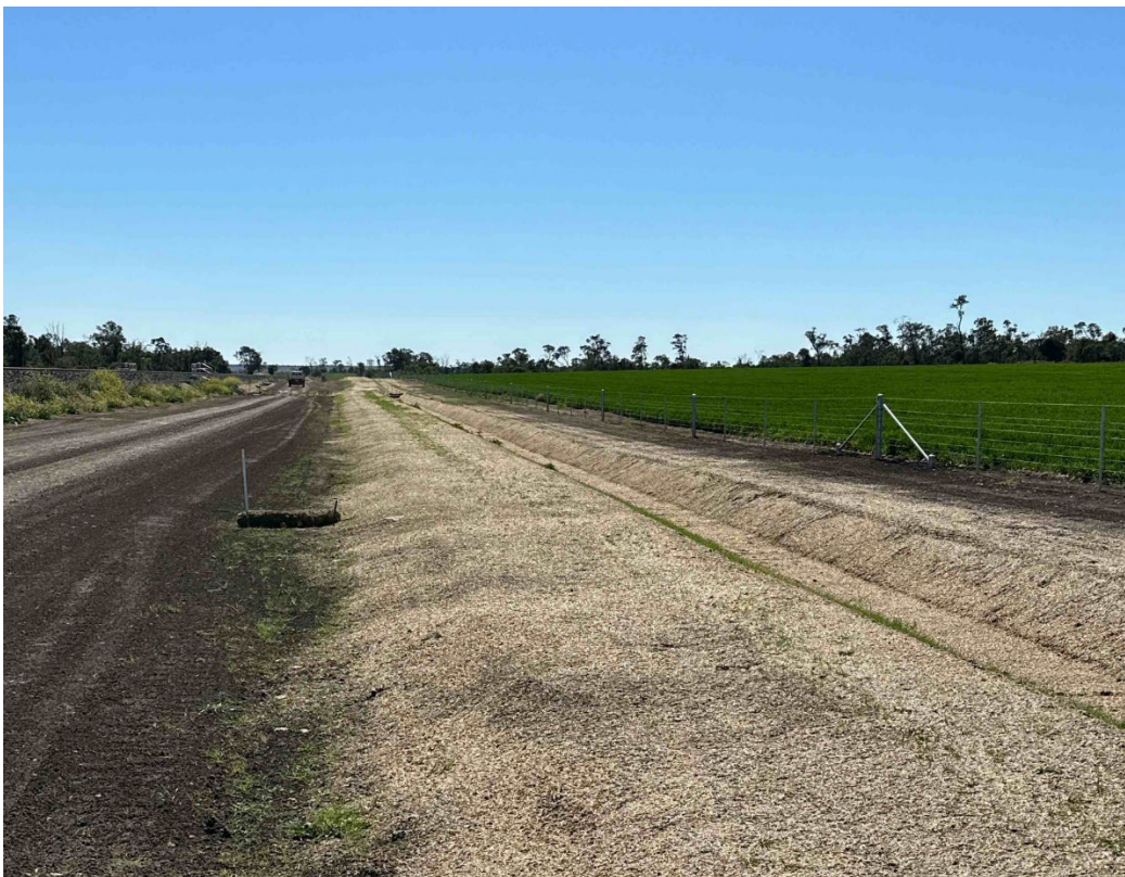
Plate 14 – Dry vegetation cover at CH746 requiring watering
