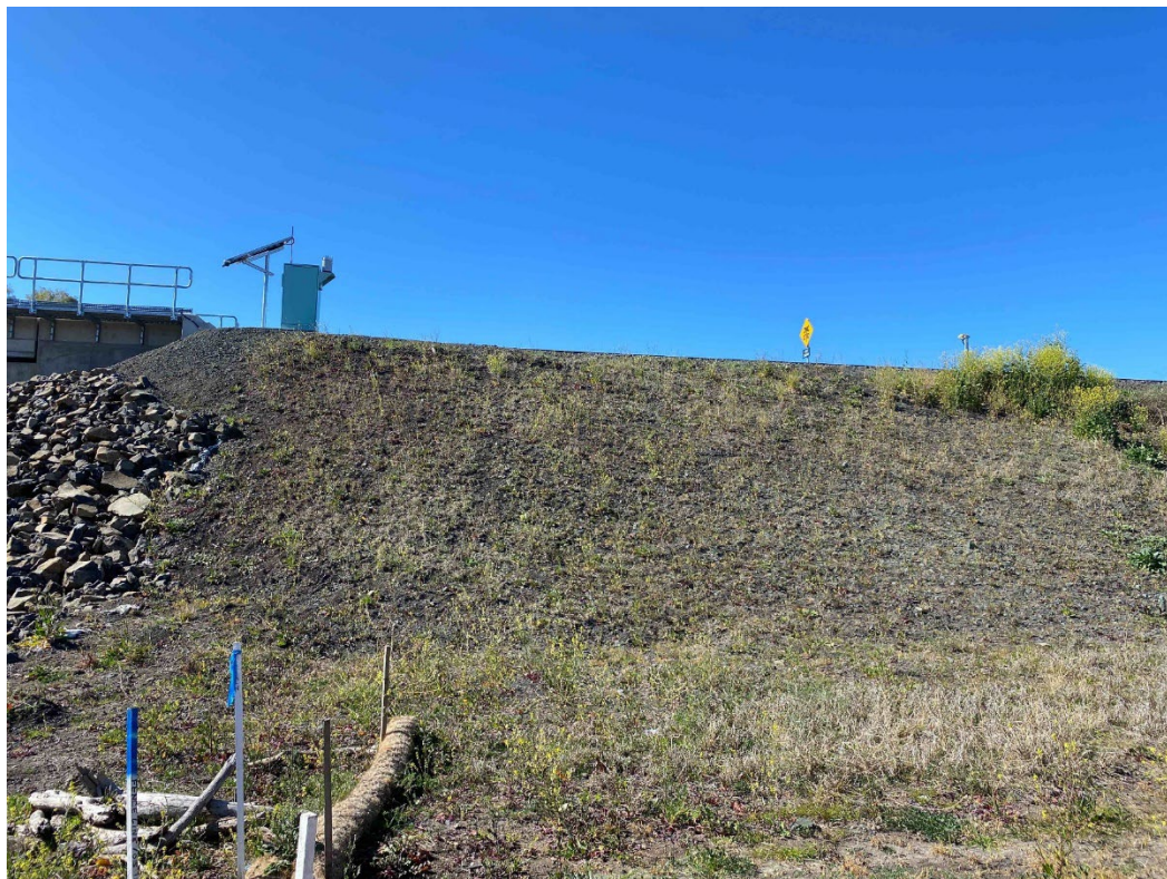
Plate 8 – Improved vegetation cover immediately south of Croppa Creek Bridge with drill seed catch evident
