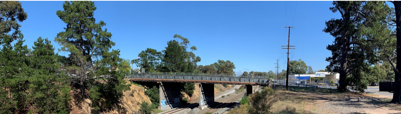
Existing Hamilton Street bridge in Broadford.
