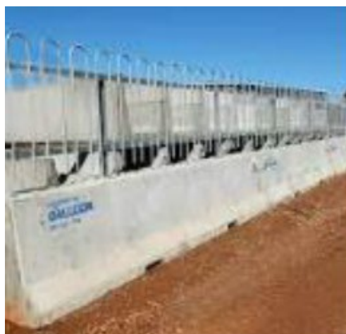
Photos 9, typical deflection screen which could be used between The Shed and the track to prevent impact near ground level
