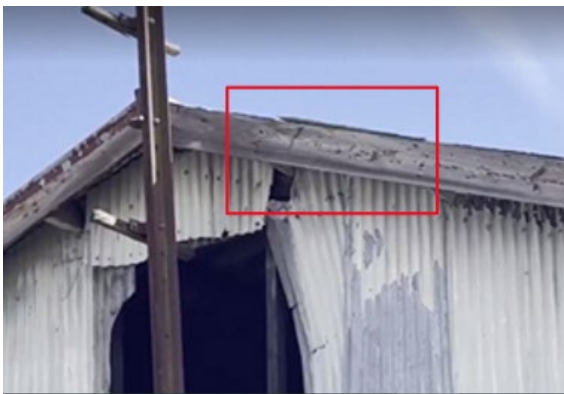
Photos 7 & 8, showing movement of roof sheeting during inspection
