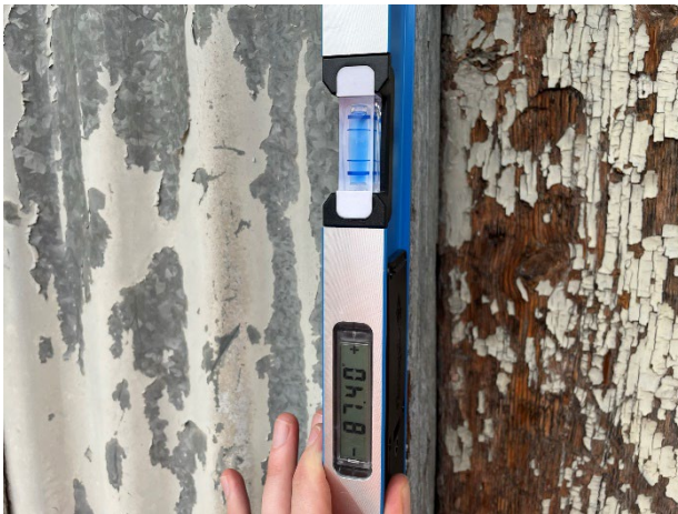
Photo: Previous incline at Downside wall (July 2023)
