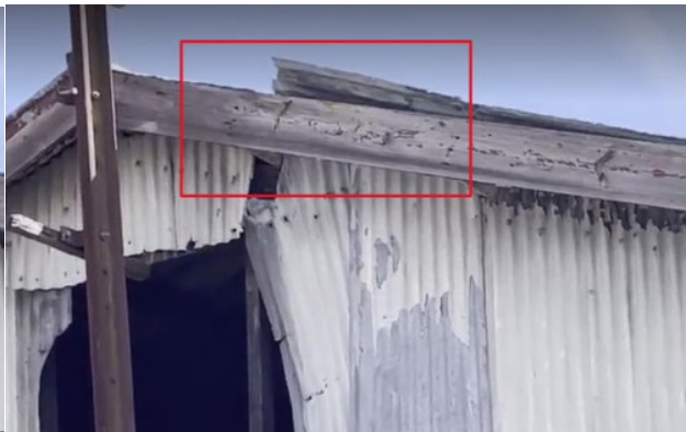
Photos 7 & 8, showing movement of roof sheeting during inspection
