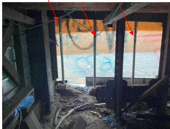
Photo 1: Steel Propping Installed
