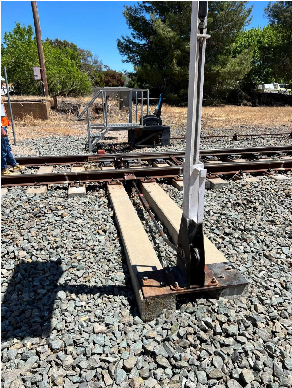
Figure 5: View to the west of the signalling assets.
