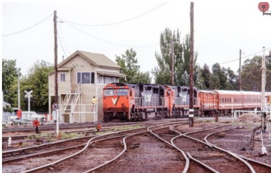
Figure 12: View of Signal Hut A in 1990. Source: Flickr.
