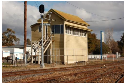
Figure 13: View of Signal Hut A in 2007. Source: vigsig.net.
