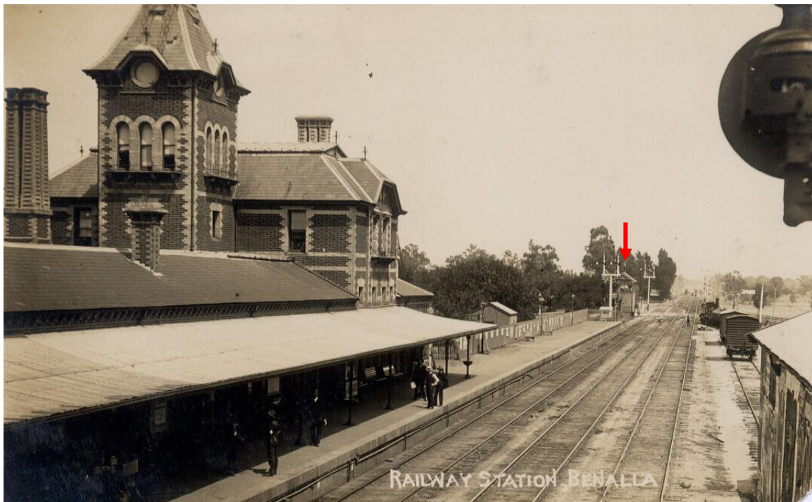
Figure 8: View of the Benalla Railway Station in the 1910s, note Signal Hut A indicated in red. Source: Flickr.
