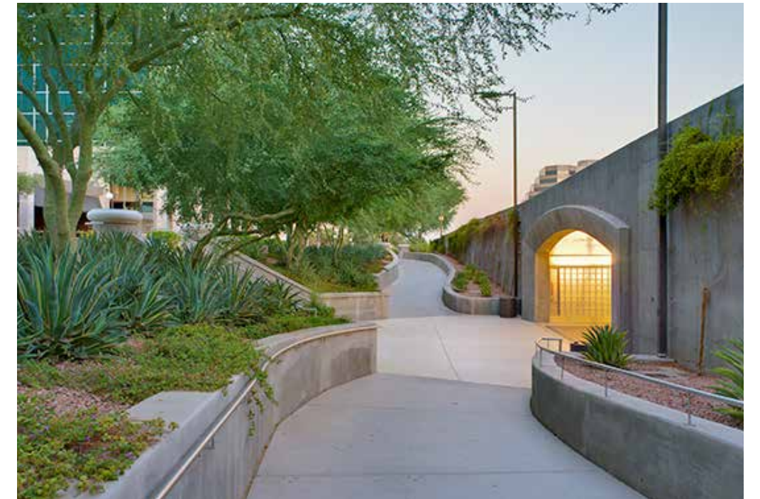
Figure 17 : Camelback pedestrian underpass, Phoenix Arizona. Landscaped embankments, clear sightlines and warm ambient lighting enhance amenity and safety of the underpass environment, especially at night.
