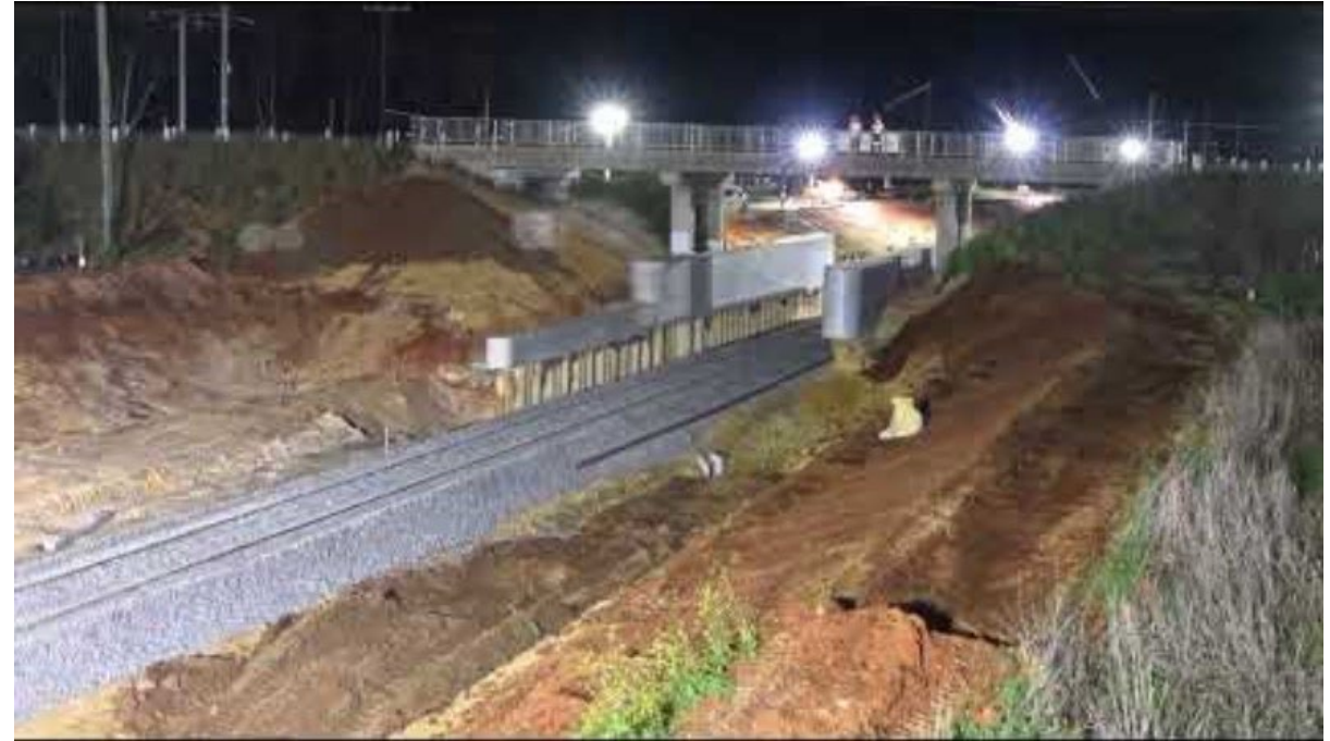
Our work: Wyndham Avenue bridge track lower at Forbes, NSW – September 2024
