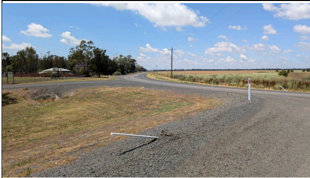
Buckie Road, Croppa Creek – View of raised road from Level crossing culvert structure to Principal's house.
