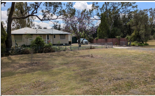
Croppa Creek Public School Principal's house – note garage on right with floor slab on ground and on piers with suspended floor.
