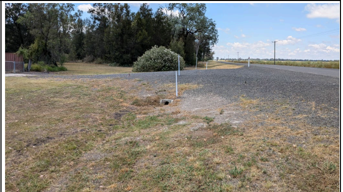
Croppa Creek Public School Principal's house driveway from Buckie Road – note difference in level from Buckie Road.
