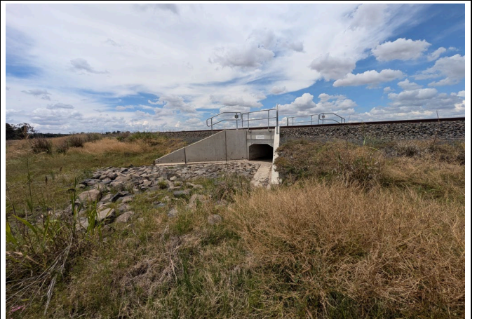
North of Boonery Park Rd – View northeast of 745.430 scour area within Pearlman Property with same suspect mound seen on the right diverting flow to culvert.
