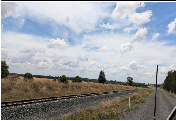
North of Boonery Park Rd, North Star – View north with new berms along alignment well vegetated.
