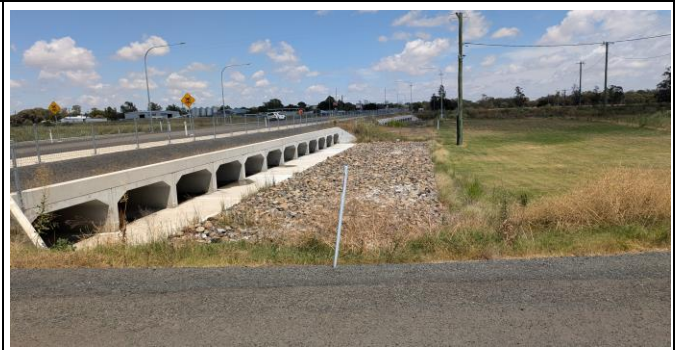
Buckie Road, Croppa Creek – View west of level crossing culvert structure.
