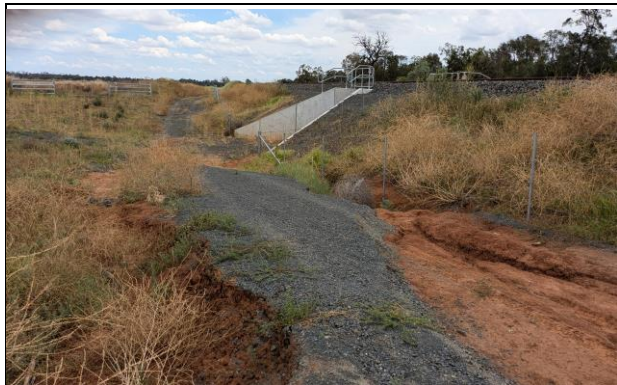
North of Boonery Park Rd - 745.879 significant scour of track access road rendering it inaccessible / unusable
