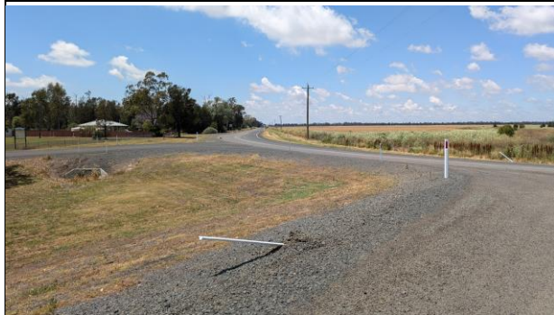
Buckie Road, Croppa Creek – View of raised road from Level crossing culvert structure to Principal's house.
