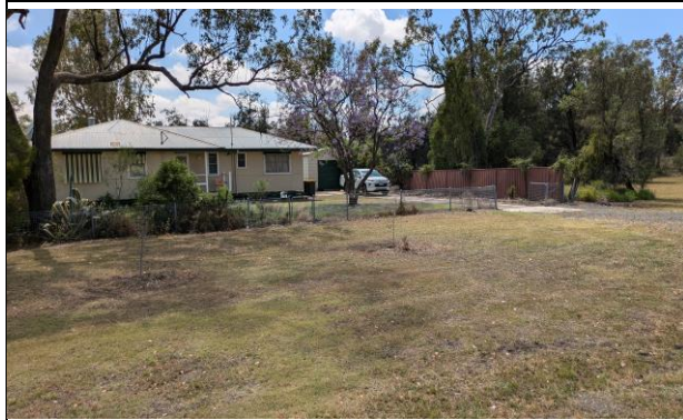
Croppa creek Public School Principal's house – note garage on right with floor slab on ground and on piers with suspended floor.
