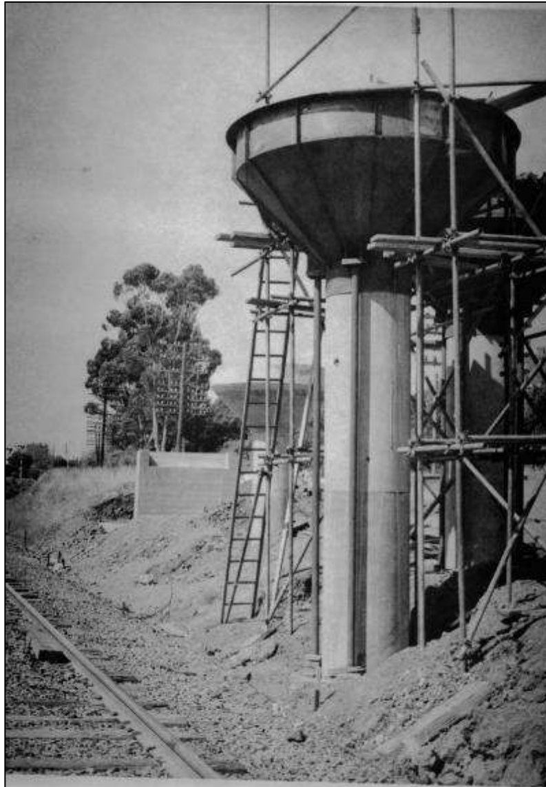
Figure 6-4: Construction of cast concrete column capitals. Source: Geoff Haddon.
