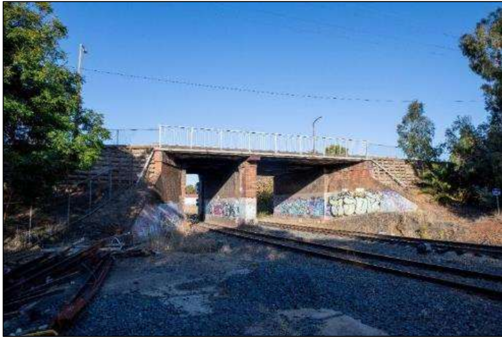
Figure 6-15: Edmondson Street Bridge brick abutments. Source: OzArk 2024.
