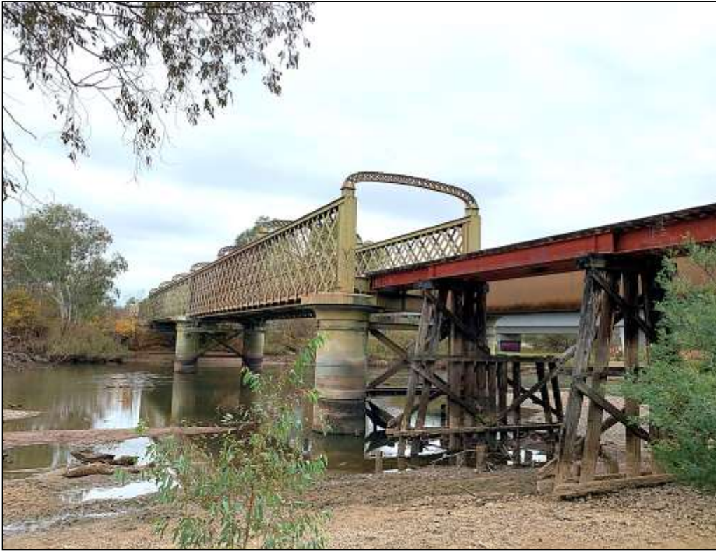
View of Murray River Rail Bridge showing the steel lattice work, horizontal bracing and various stages of construction.
