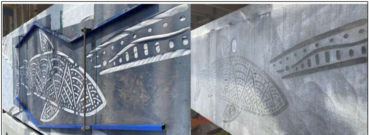
Figure 10-20: Precast deck units sandblasted with Ngarrindjeri characters and Clan motifs. Source: Government of South Australia.
