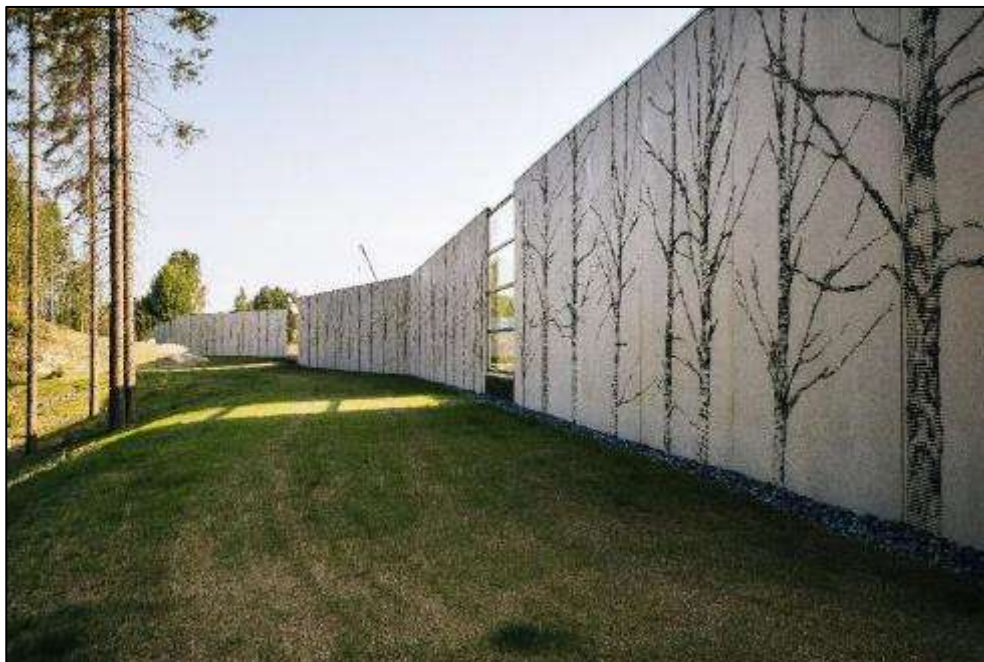
Figure 10-33: Birch trees engraved into concrete noise walls, with transparent windows. Source: Ramboll, Finland.
