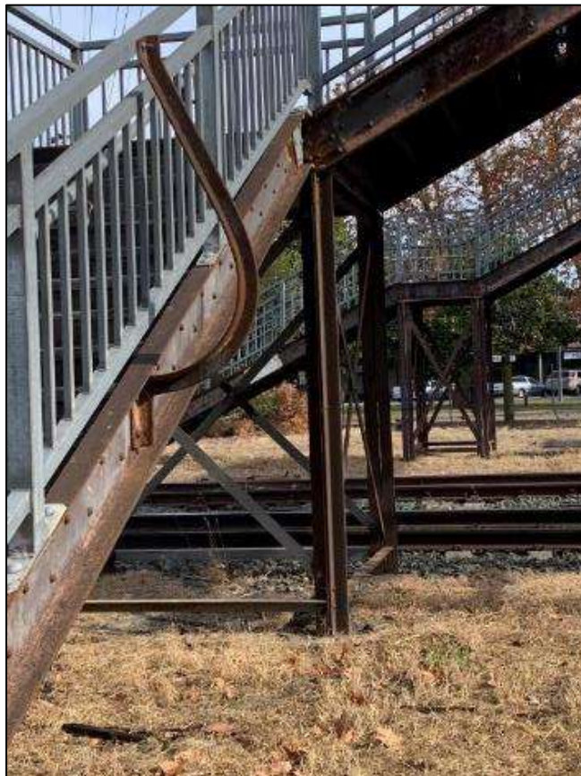
Figure 5-3: Details of curved lateral braces and lightweight structural elements. Source: OzArk 2024.
