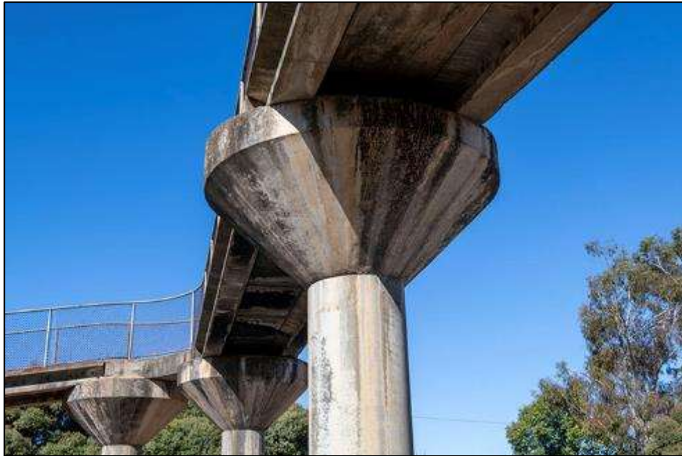
Figure 6-6: Cone-shaped column capitals. Source: OzArk 2024.
