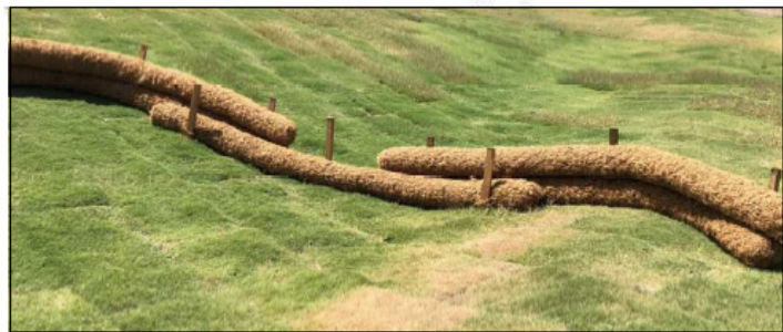
COIR LOG SEDIMENT TRAP
