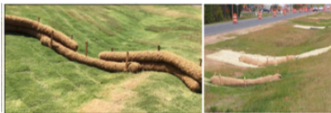
Coir log sediment trap and coir log velocity control in drainage lines
