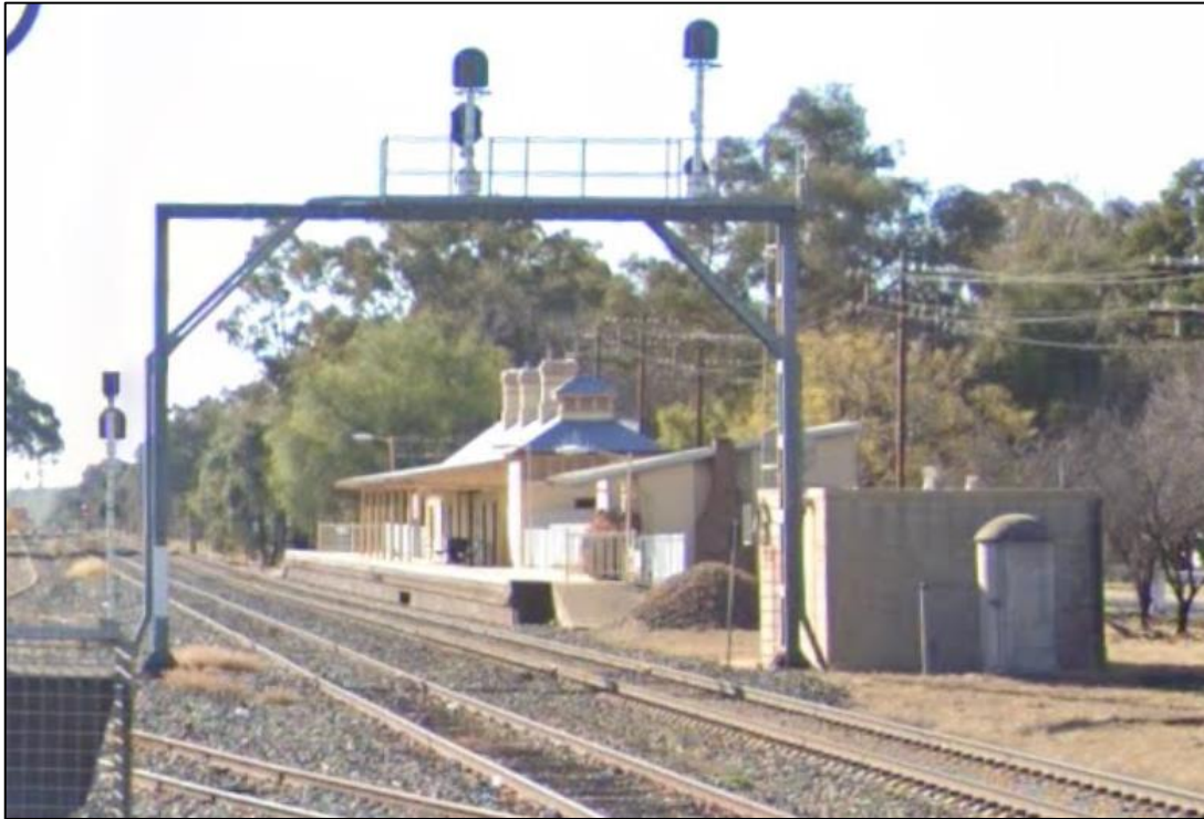
Figure 6-2: East view of the existing gantry approved for modification. The post-1980s relay room is to the left (north) of the gantry (source: Google Earth).
