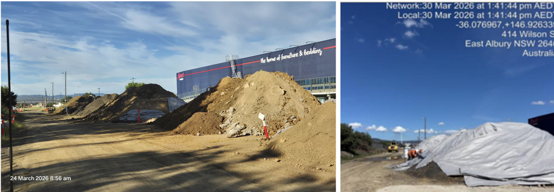
Figure 1. Riverina Stockpile area (stockpile coverage)– (24/03/26 left (ER inspection), 30/03/2026 right (MR))
