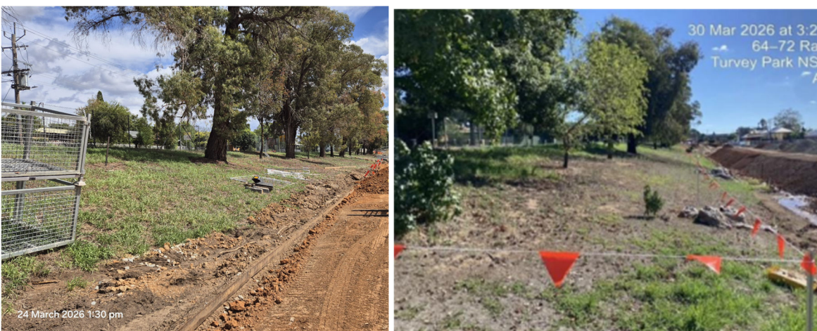
Figure 3. Wagga Yard (tree protection / delineation) (24/03/26 left (ER inspection), 30/03/2026 right (MR))
