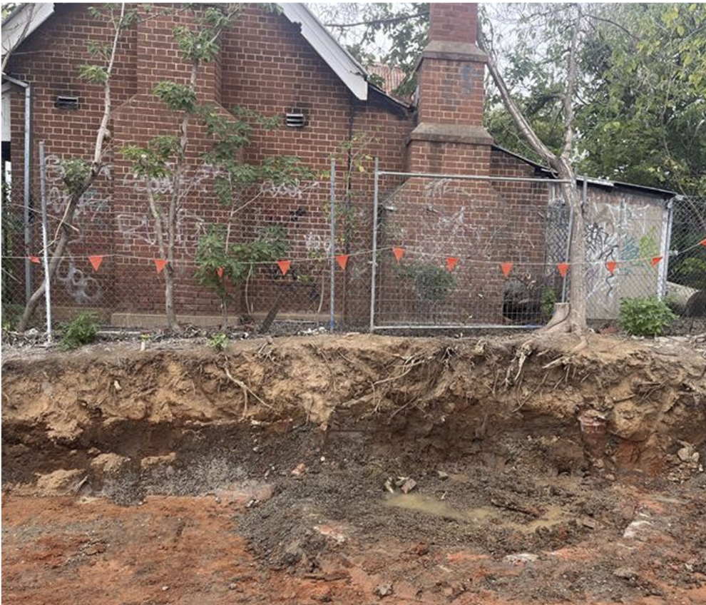
Image of unexpected find (circular brick work on the ground) provided by MR
