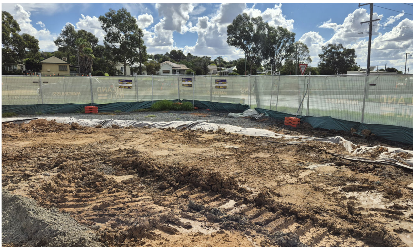
Figure 5. Wrights Oval compound (bund to be raised, and rock filter dam installation as per PESCP in progress) (24/03/26 ER inspection)
