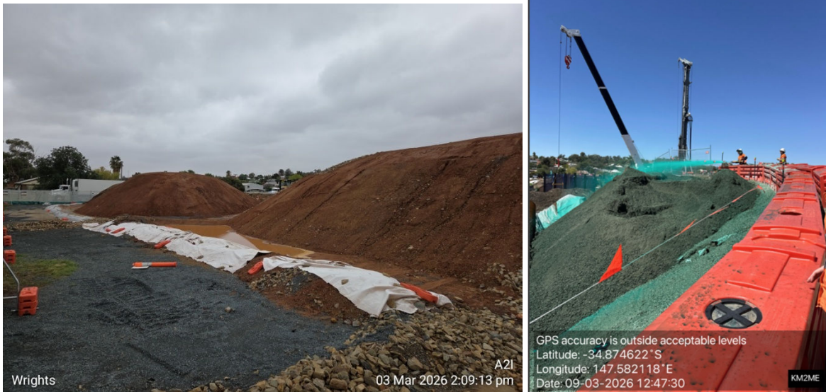
Figure 4. Wrights oval compound (stockpile stabilisation) (3/03/26 left (ER inspection), 9/03/2026 right (MR))
