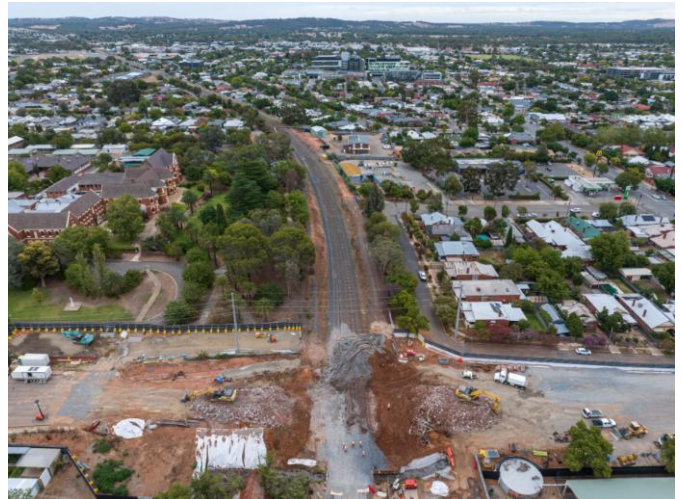
Photo: Edmondson bridge removed.
