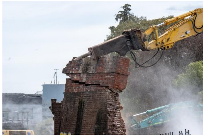
Photo: Edmondson bridge demolition.
