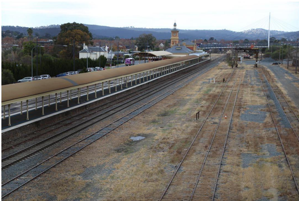
Figure 1. Overview of the Albury Railway Station and Yard taken from the southern pedestrian overpass looking north. Source: Extent Heritage 2024.
