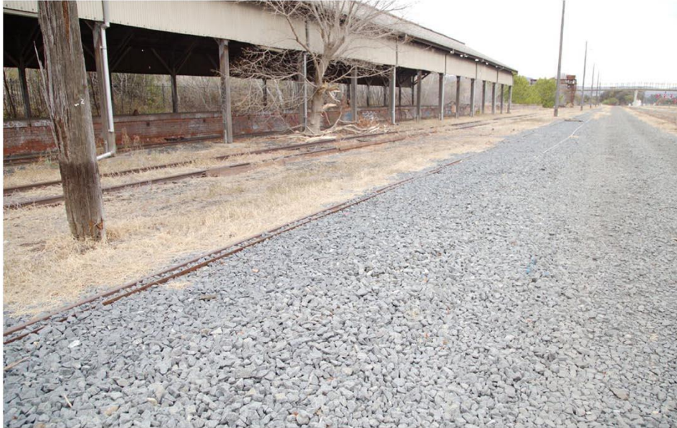
Figure 42. View of Track 5 facing south showing section covered with ballast. Source: Extent Heritage.
