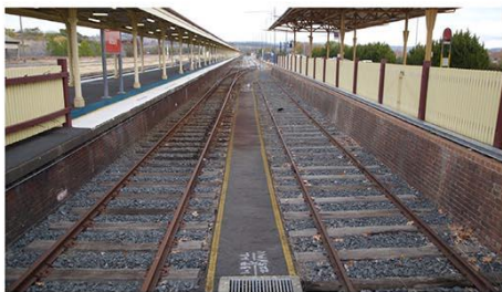
Figure 47. View south along cripple siding showing Broad Gauge track to the right and Standard Gauge to the left. Source: Extent Heritage.
