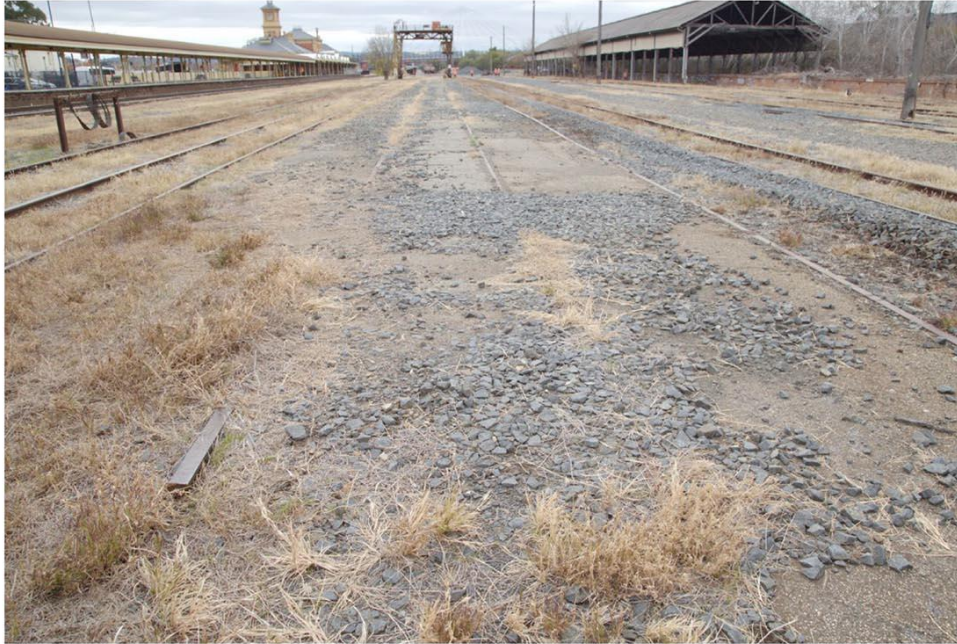
Figure 45. View of Track 3 facing north. Source: Extent Heritage.
