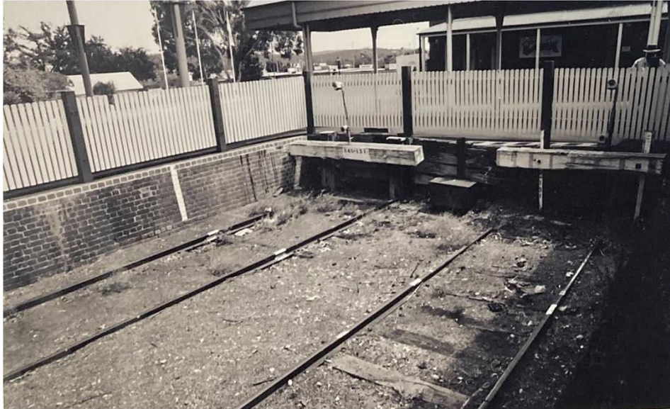
Figure 24. View of northern end of Broad Gauge platform 2 with buffer stops. Source: O.H.M Consultants, 2009.
