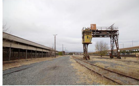
Figure 34. View of former Transshipment Shed and gantry crane within the railway yard facing south. Source: Extent Heritage.
