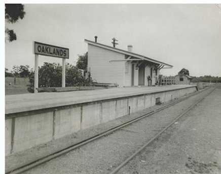
Figure 26. Dual gauge railway line at Oaklands Station, 1960. Source: Weston Langford Railway Photography n.d.
