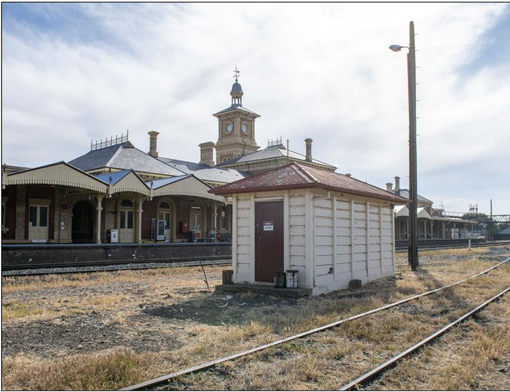
View of Signal Box 1A, part of the Albury Railway Station and Yard Group (OzArk: May 2024).
