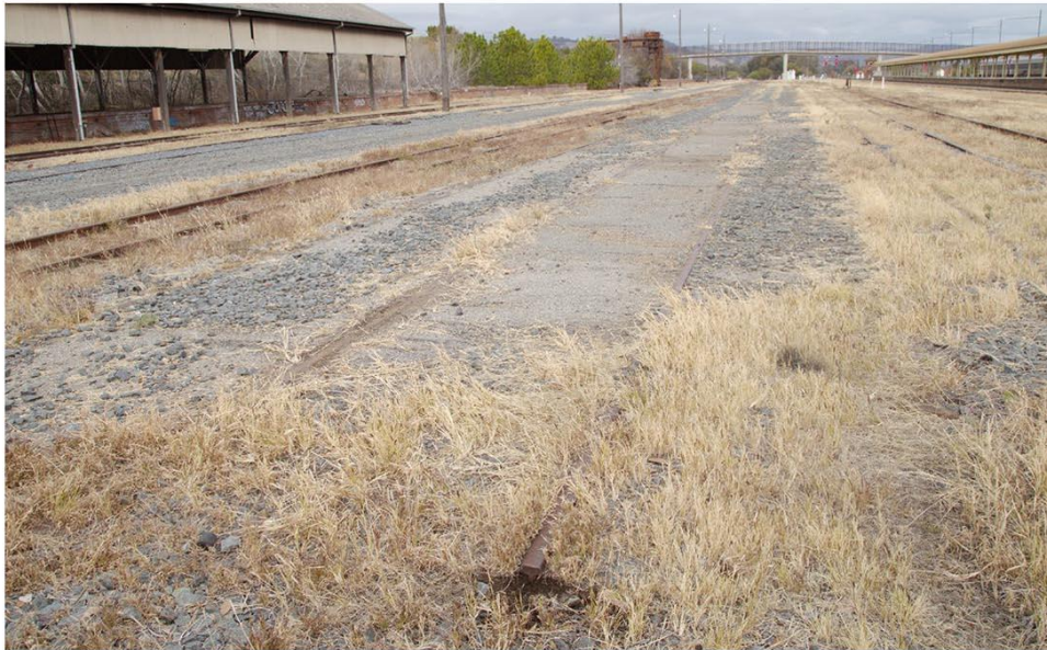
Figure 44. View of Track 3 facing south. Source: Extent Heritage.
