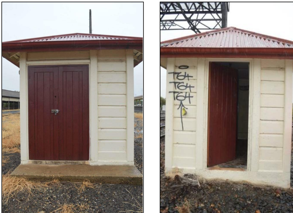
Figure 2-7: Albury Signal Box 1A (left) and Albury Signal Box 1B (right) (Source: GML Heritage 2022: 4).
