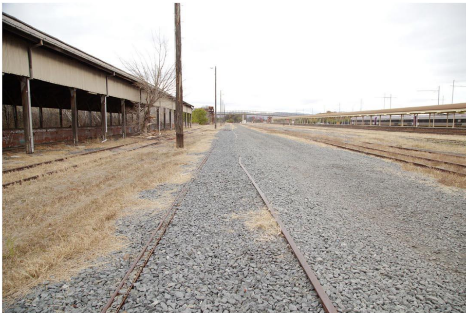
Figure 39. View south along Track 5 showing the easternmost rail to the left which is on its side and the western rail to the right which is bent. Source: Extent Heritage.
