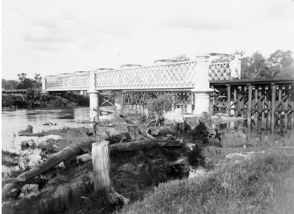
Figure 9. Albury Bridge connecting Victoria and NSW. Source: Museums of History NSW, State Archives, NRS 4481-3.
