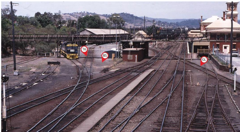
Figure 21. c.1980s photograph of the Yard viewed south from the northern pedestrian bridge. The Track 3 and 5 alignments are obscured from view in this photograph. However, other key elements including the Goods Line (GL), Transshipping line buffer stop (BS), and Track 6 (T6) are visible and labelled accordingly. Source: GML 2023, 6, with Extent Heritage overlay.
