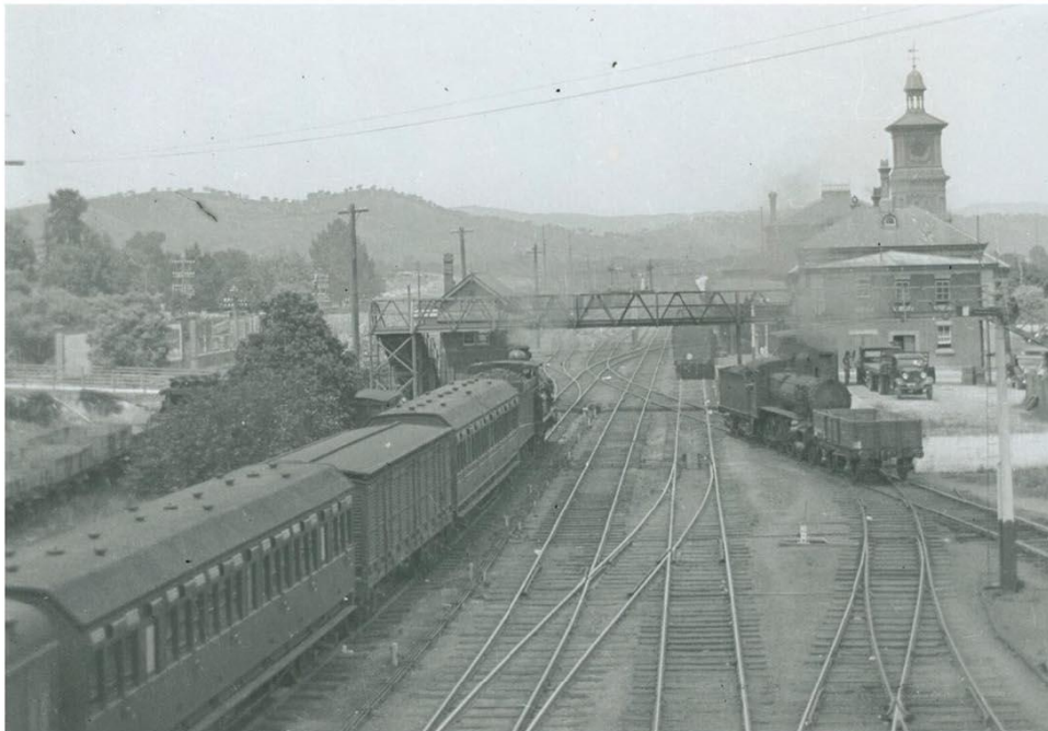
Figure 8. Albury Railway Station c.1920, with broad-gauge locomotive and truck on right and Standard Gauge locomotive and track on the left. Source: National Library of Australia, Bib ID 3422852.
