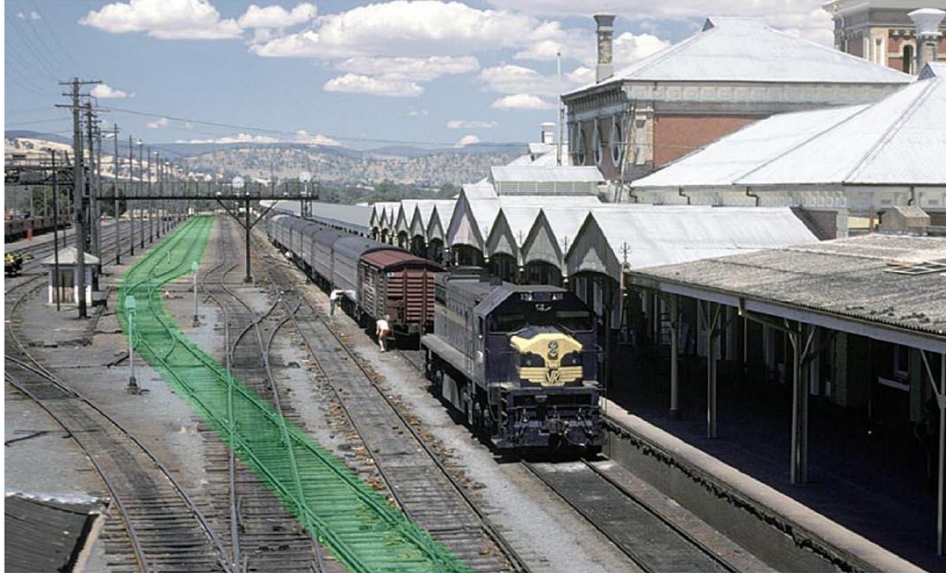
Figure 20. 1981 photograph of the railway corridor looking south from the pedestrian footbridge. The photograph shows the presence of the Broad Gauge Goods Line (highlighted in green) remaining in situ at the Yard during this period. Source: Victorian Railways, https://www.victorianrailways.net/photogallery/northeast/albury/albury.html , with Extent Heritage overlay.
