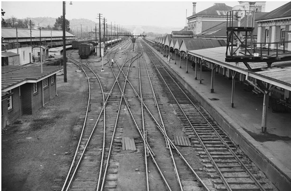
Figure 13. View along rail yard in front of station facing south taken from the steel footbridge located adjacent to the signal box. Source: Museums of History NSW, State Archives NRS-22474-2-4-S2603.
