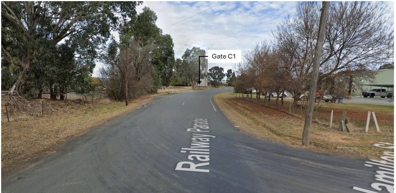
FIGURE 21: SOUTHBOUND VIEW APPROACHING GATE C1 (~100M FROM ACCESS POINT)
