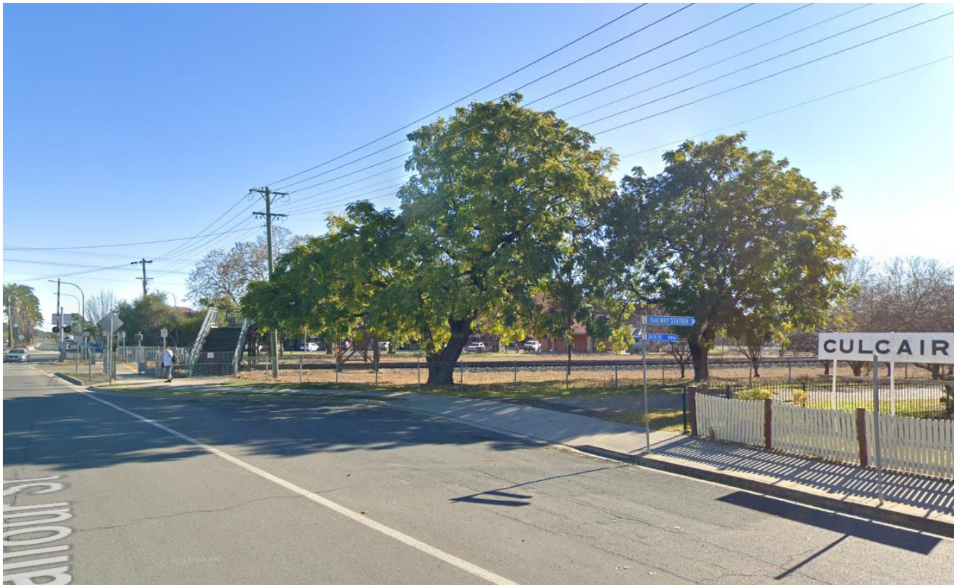
FIGURE 27: GATE C3 – EXISTING ACCESS OFF BALFOUR STREET (OLYMPIC HIGHWAY)
