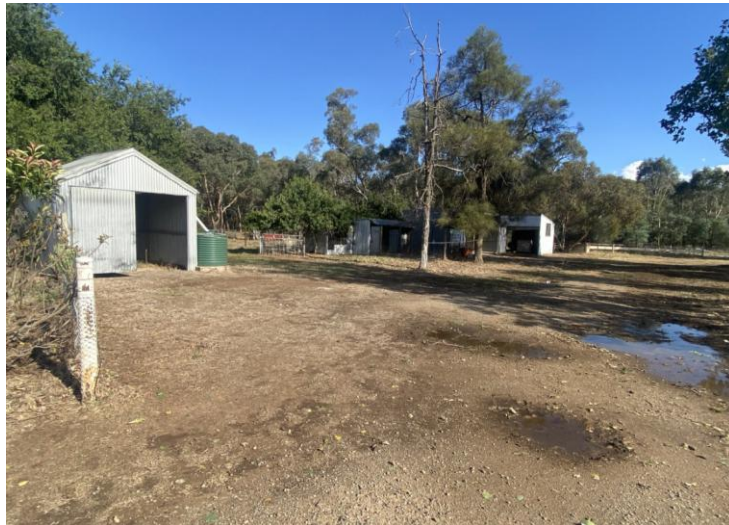
Figure 4-2 Existing sheds to be utilised for storage
