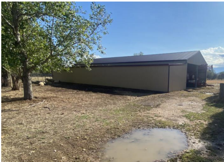
Figure 4-3 Existing sheds to be utilised for storage
