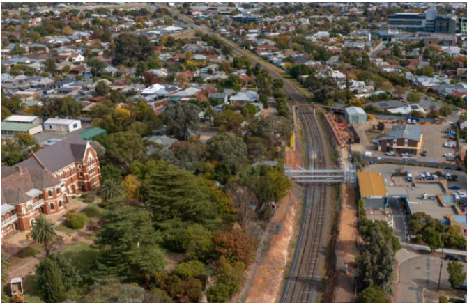
Photo: Cassidy temporary scaffold bridge mid construction May 2026
