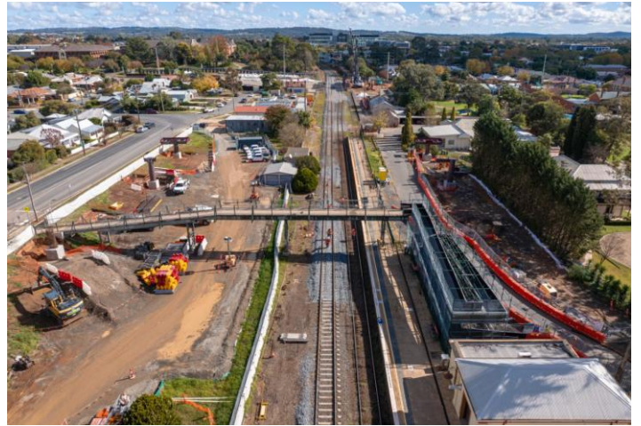
Photo: Wagga Wagga Station site works
