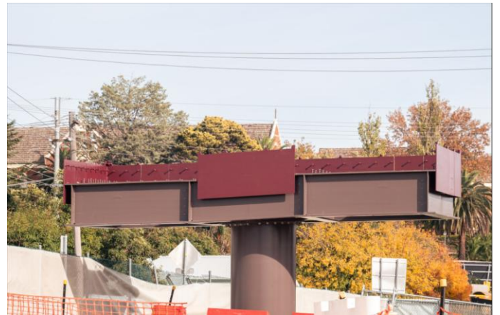
Photo new Mothers bridge ramp columns May 2026
