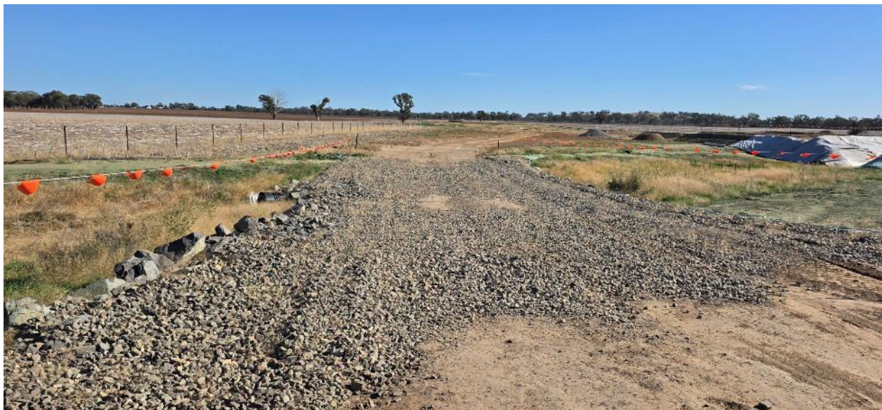
Temporary piped crossing for fish passage installed at Powder Horn Creek.
