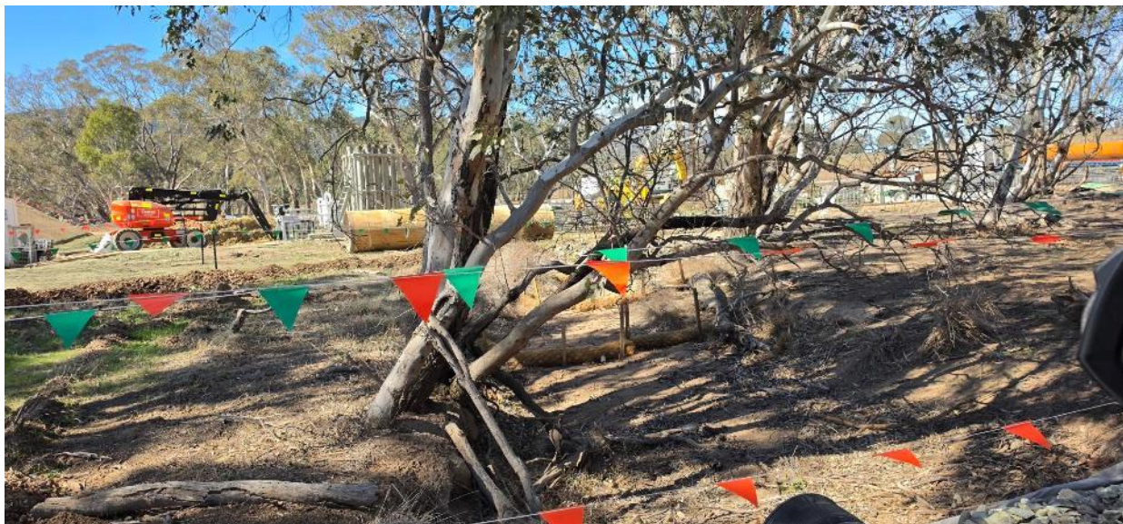
Flagging installed for construction and environmental sensitive area at Run Boundary Creek.
