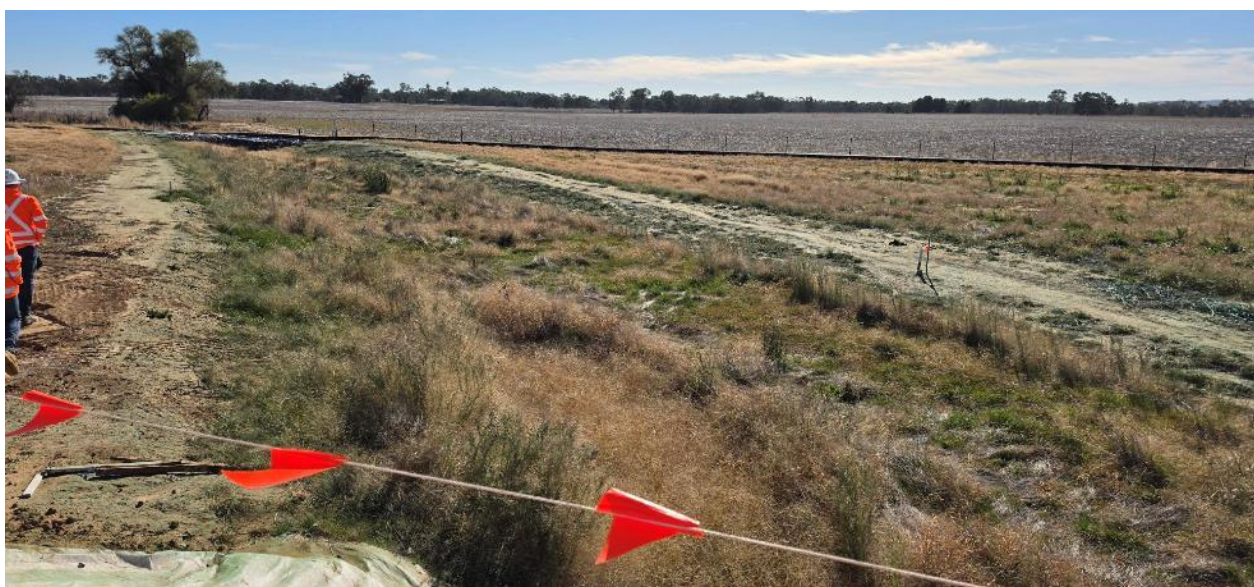
Existing ground cover / vegetation noted throughout the creek with exposed areas stabilised with polymer binder.
