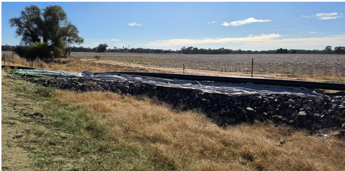
Rock filter dam installed at Powder Horn Creek.
