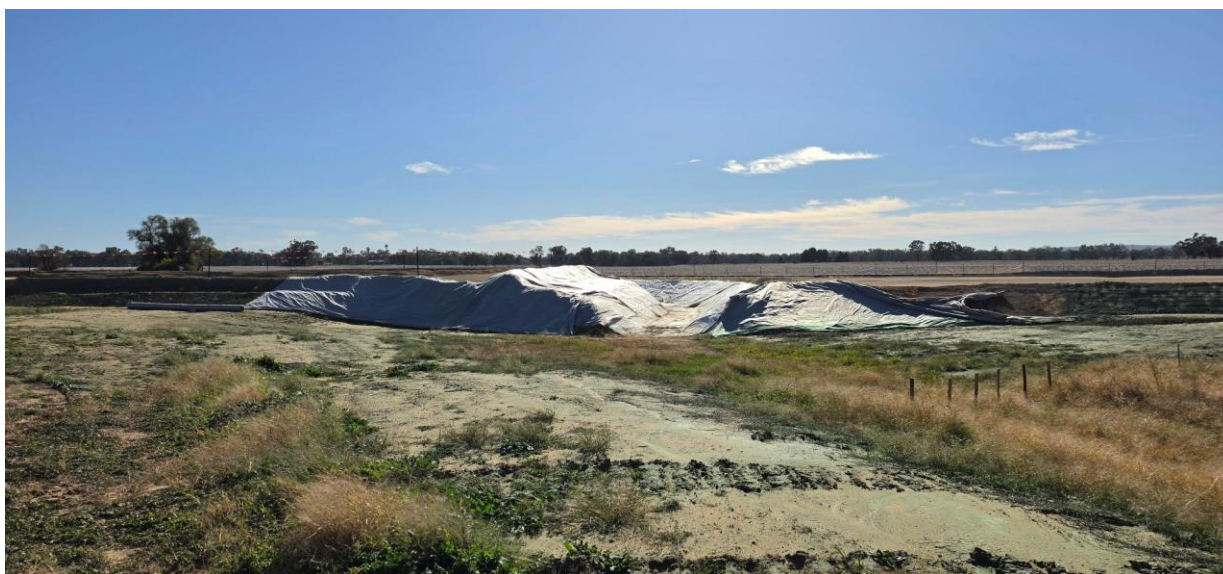
Clean water diversion installed and lined with geofabric at Powder Horn Creek.
