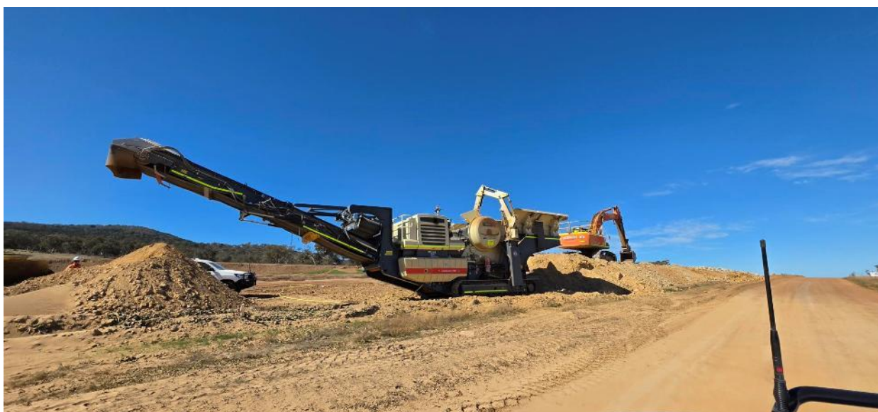
Mobile crusher in operation processing material for reuse.
