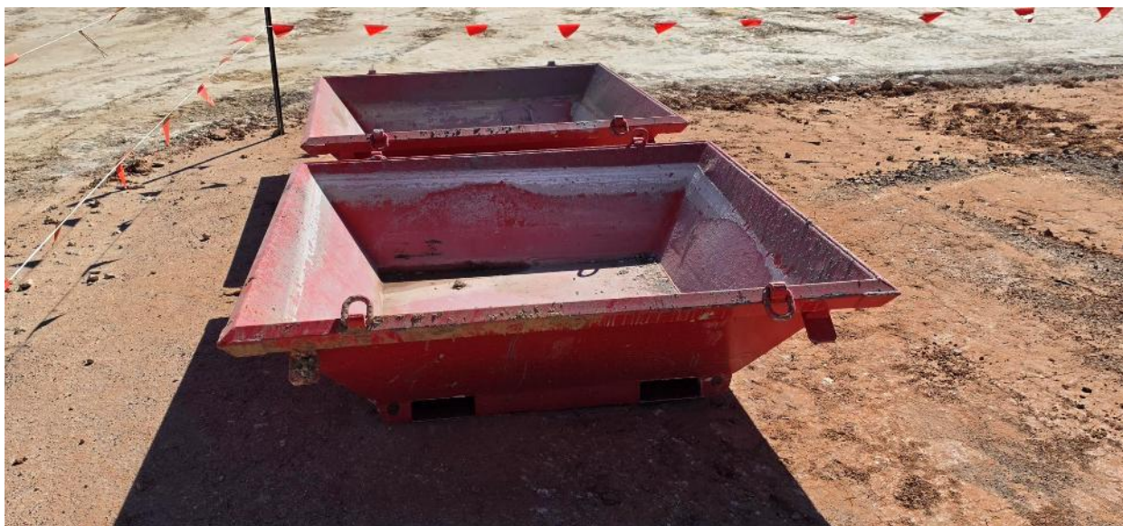
Concrete washout trays.
