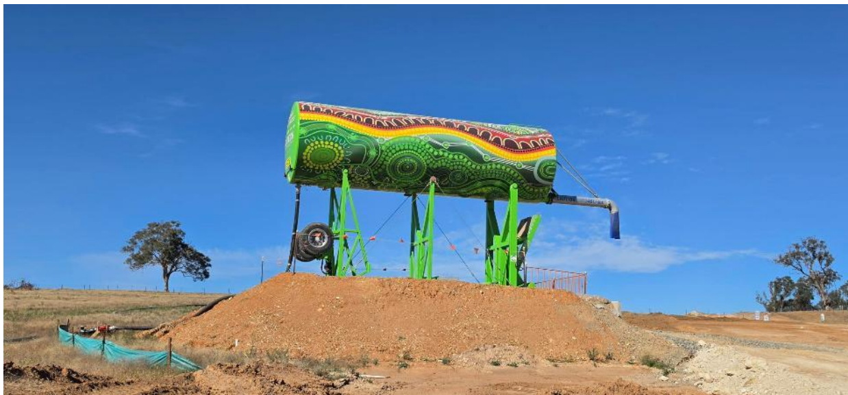
Water fill points installed along the alignment, with silt fencing in place as sediment control.
