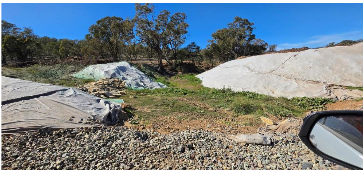
A bed level crossing installed at Unnamed Creek with batters covered with geofabric.
