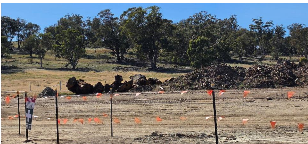
Vegetation and timber stockpiles retained on site for reuse.
