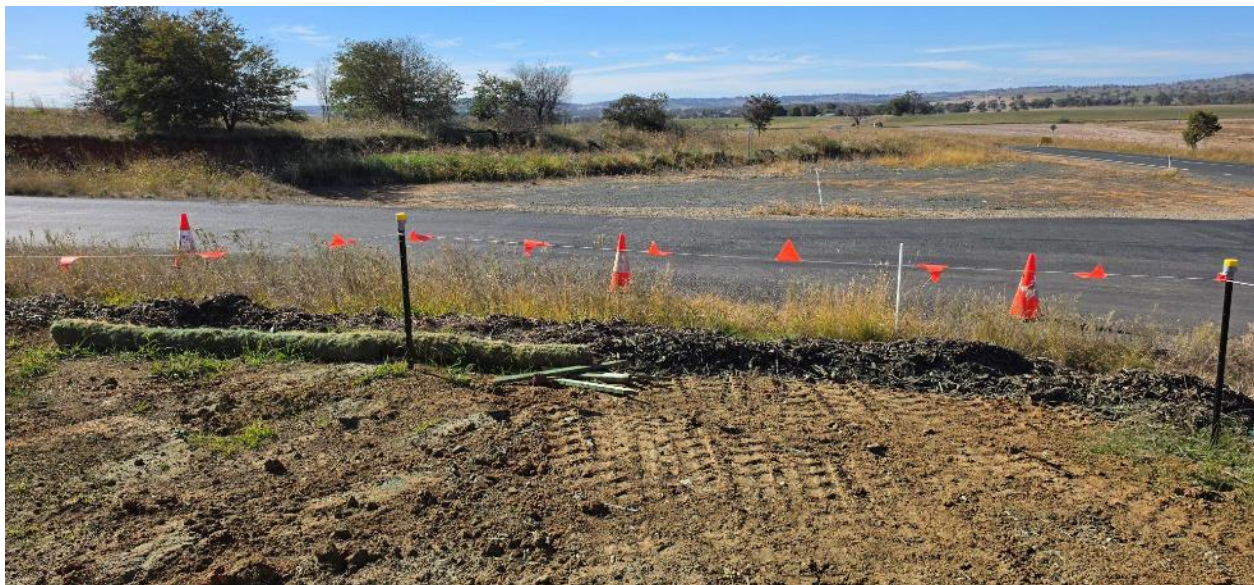
Mulch bunds installed along the verge of Dirnaseer Rd.
