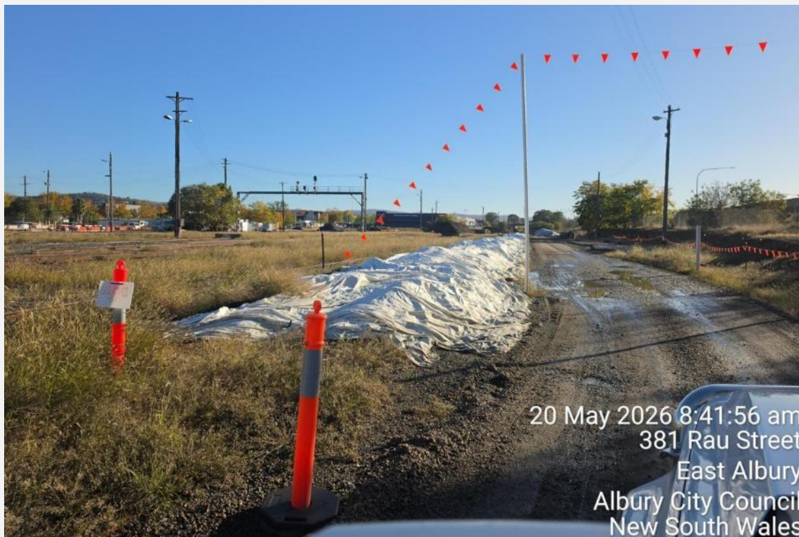
Stockpile delineated and covered with geofabric.
