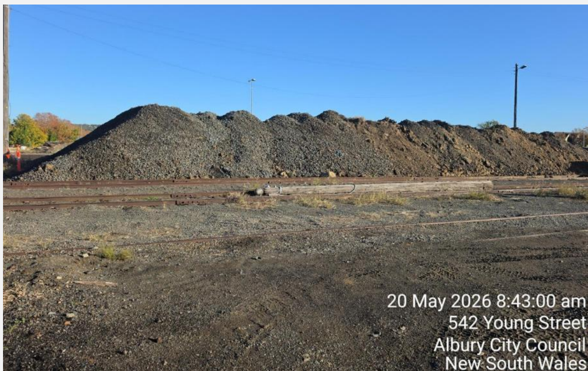
A recent stockpile generated during the May possession stored on site, pending testing results.
