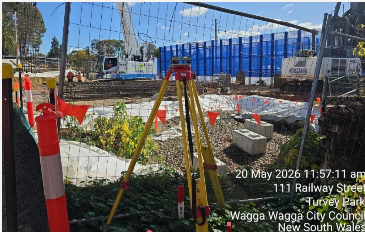
Piling works in progress with exclusion zone installed.
