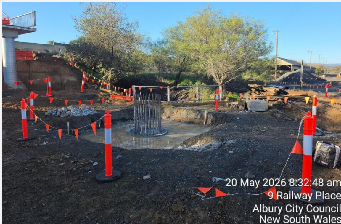
Pedestrian bridge construction in progress at Albury Station.
