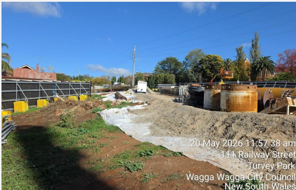
Erosion and Sediment (ERSED) controls observed to manage stormwater.
