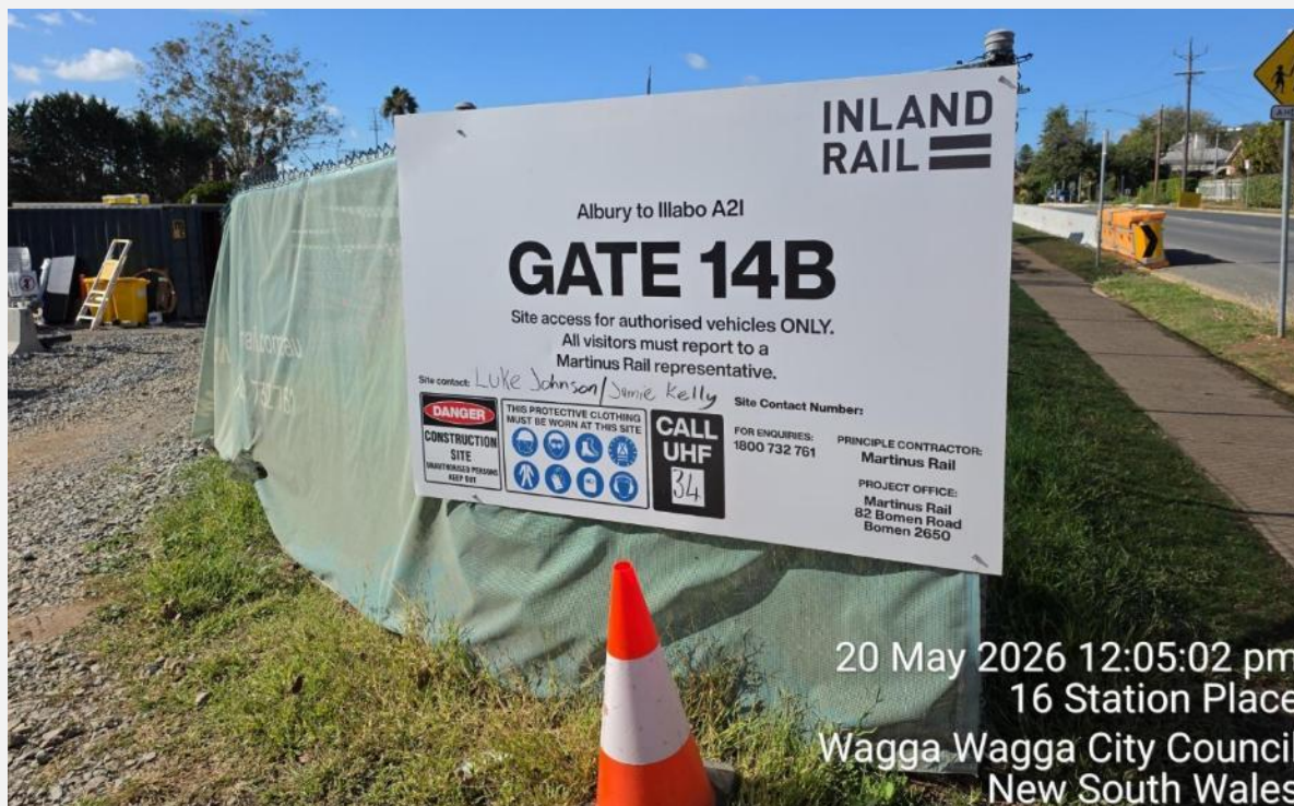
Project signage displayed on site.
