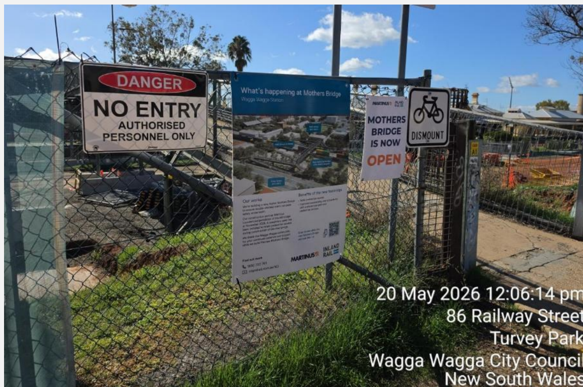
Directional signage and project information displayed at Mothers Bridge.
