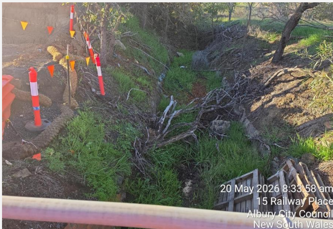
Coir logs have been installed along the waterway boundary for the pedestrian bridge works.
