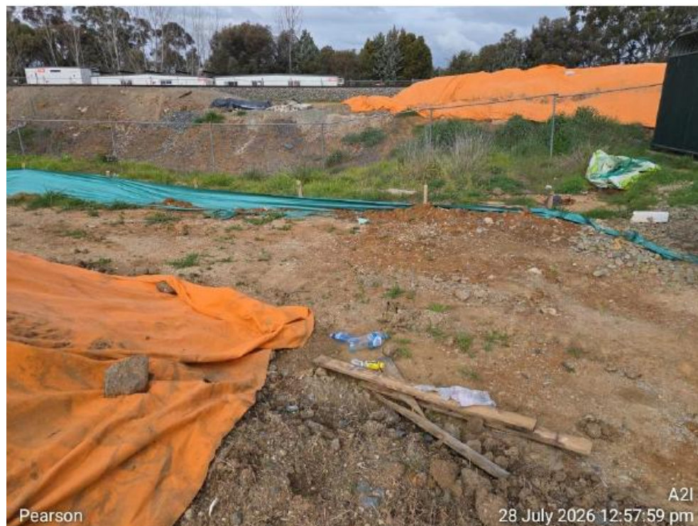
Figure 3. Pearson St – Rubbish to be removed and sediment fence to be maintained / removed (28/07/26)
