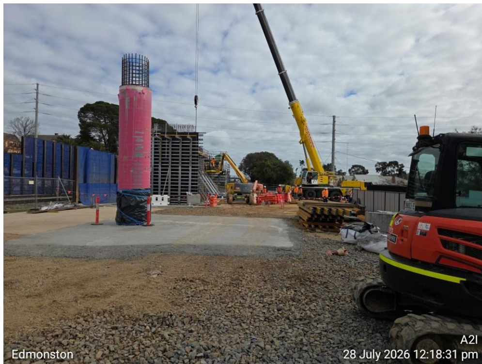
Figure 4. Edmonston St – Piling activities (28/07/26)
