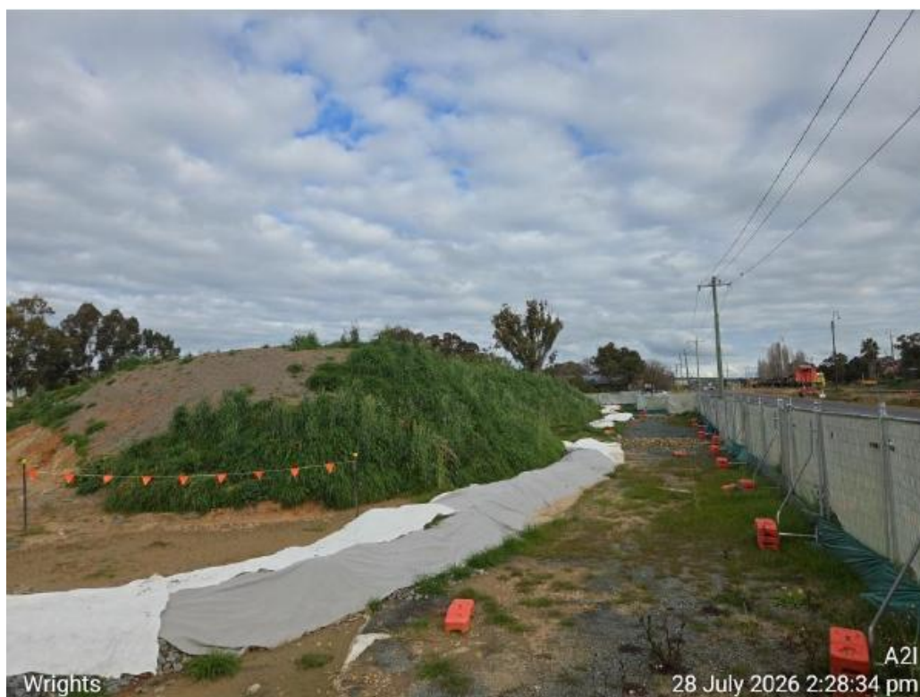
Figure 6. Wrights Compound, Junee – Establishment of groundcover on stockpile (28/07/26)
