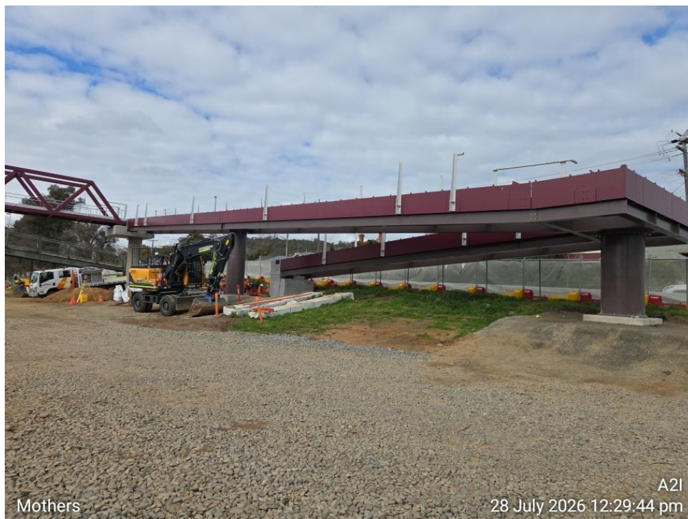
Figure 5. Mothers Bridge – Southern ramp and deck in place (28/07/26)
