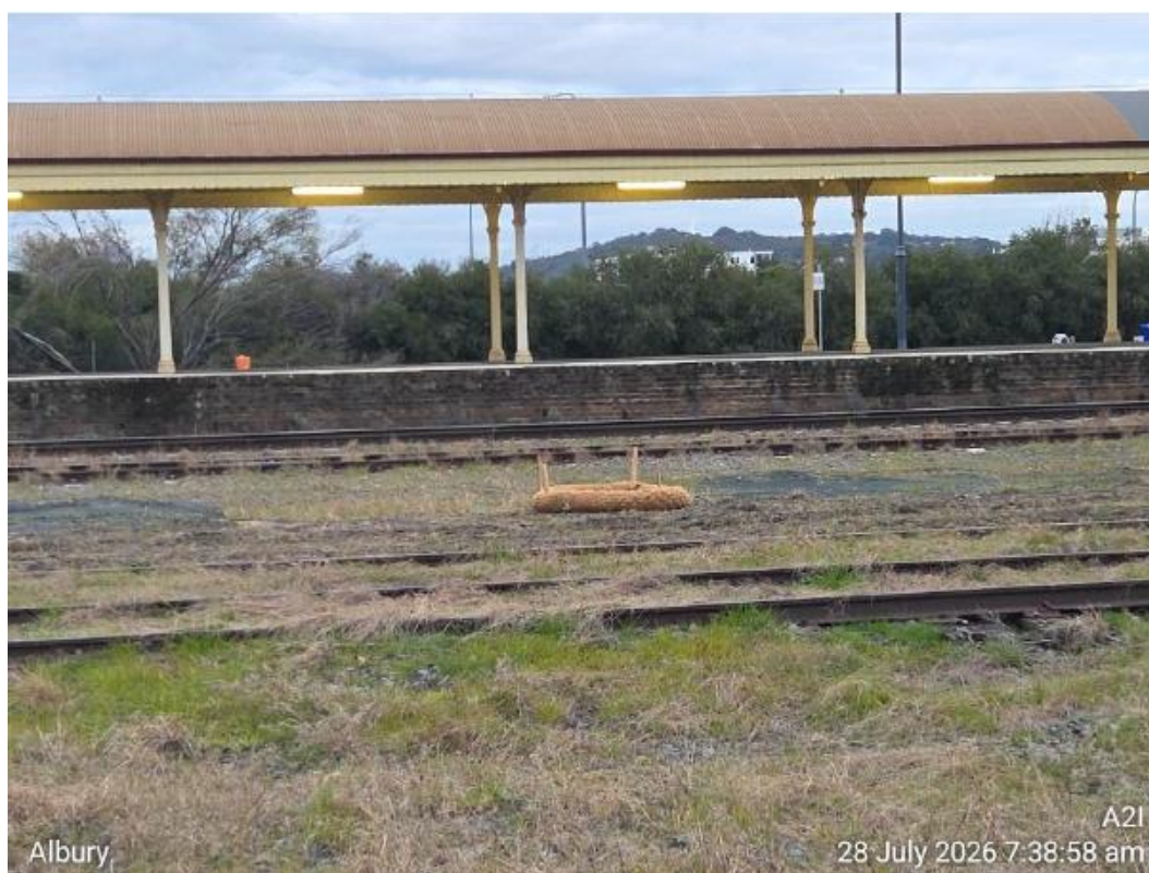
Figure 2. Riverina – pits protected with inlet filters (28/07/26)
