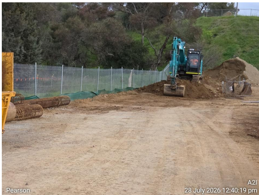
Figure 5. Pearson St – Spoil being removed (28/07/26)
